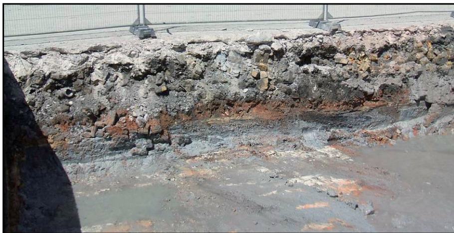
Plate 4 Area C: south-east facing section of kiln structure (south end).
