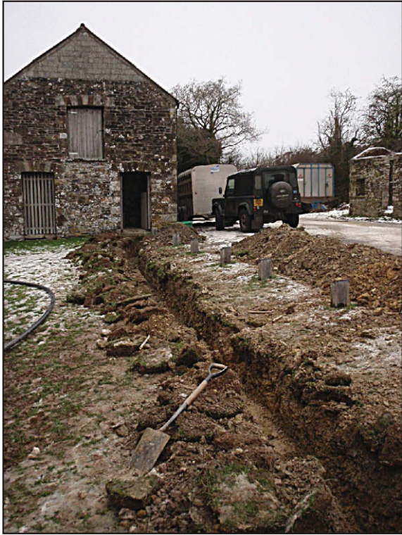
Pl. 1 General view of trenching. Looking north.
