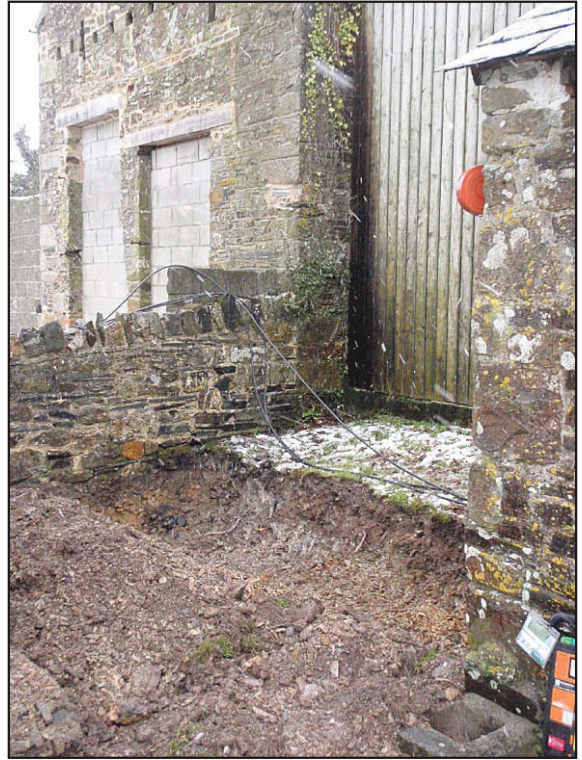
Pl. 2 General view of trenching behind barn. Looking north.
