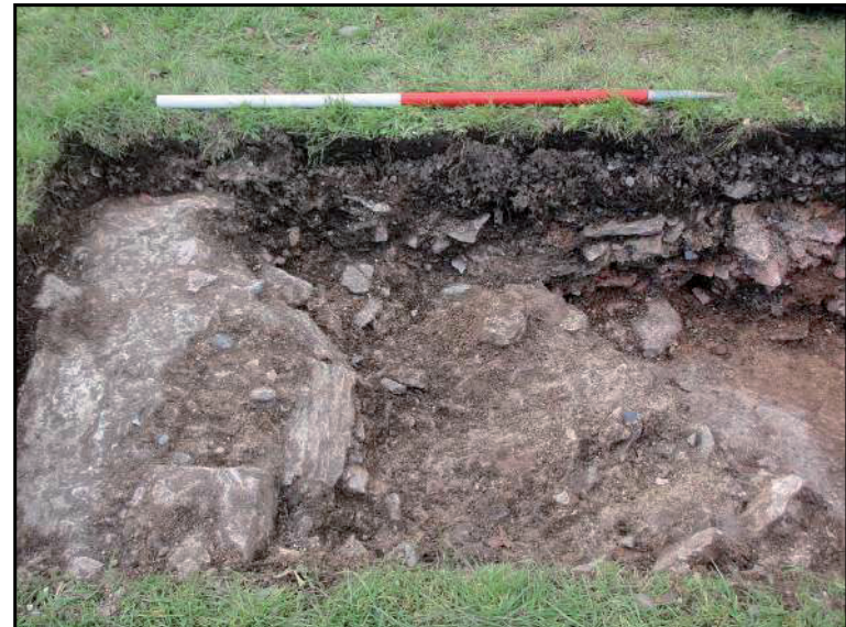
Pl. 8 Detailed view of rubble core of ravelin scarp wall and 'Barrack Office' wall. Looking west. 1m scale.
