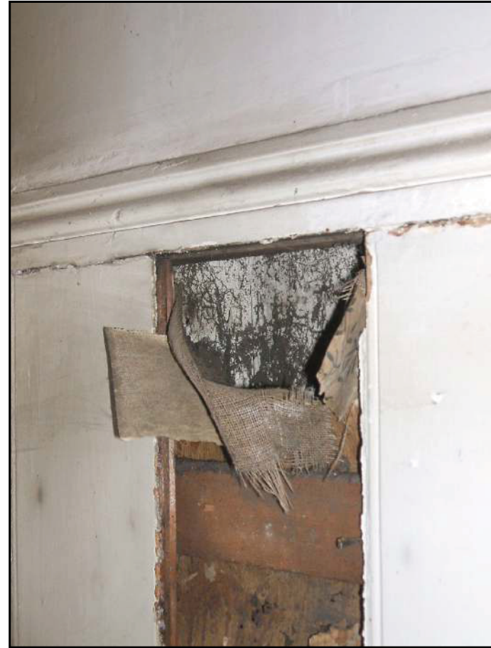
Pl. 4 57 Bampton street: plank-and-muntin screen behind later cladding, looking north-west.
