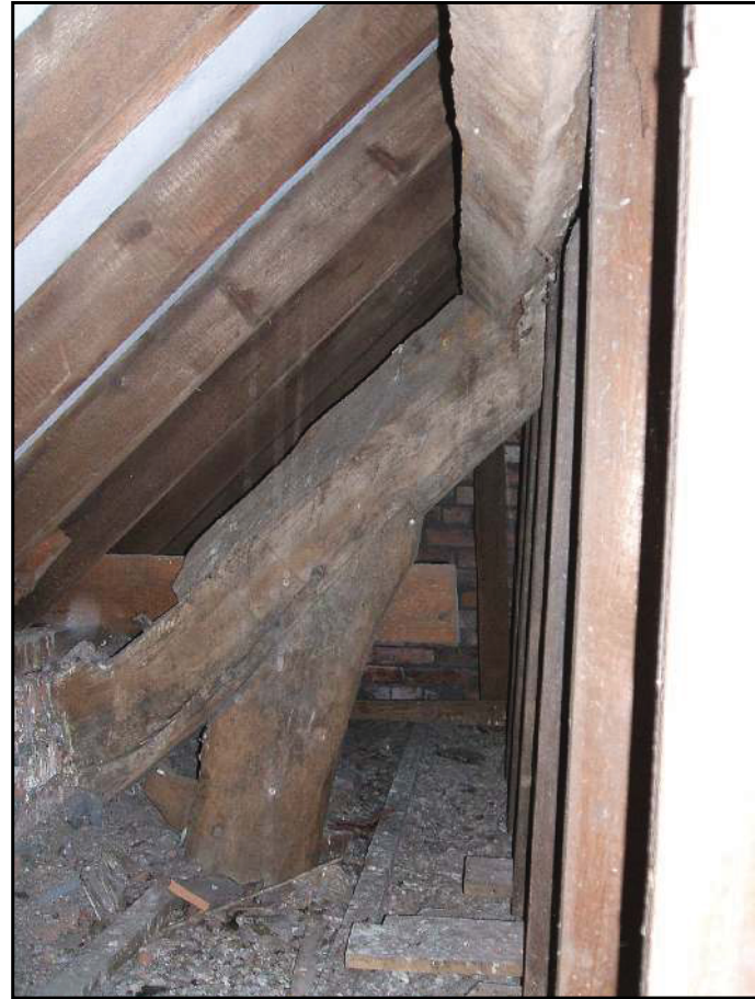
Pl. 6 Jointed-cruce truss in the southern rear wing, looking east.
