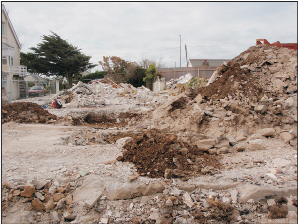
Plate 2 General view of site. Looking south.
