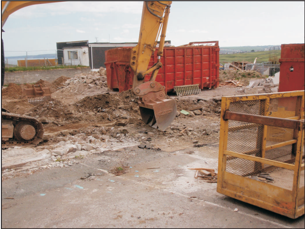
Plate 1 General view of site. Looking northeast.
