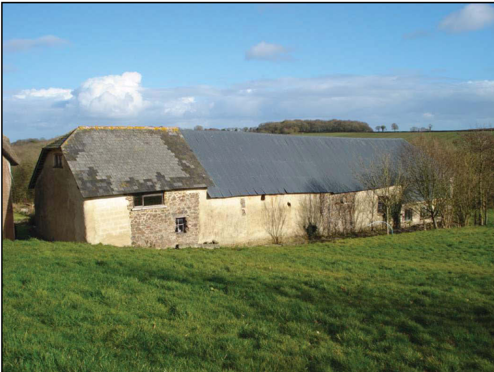
Fig. 3 General view of the farm buildings, looking south east, showing the rear elevation prior to conversion.
