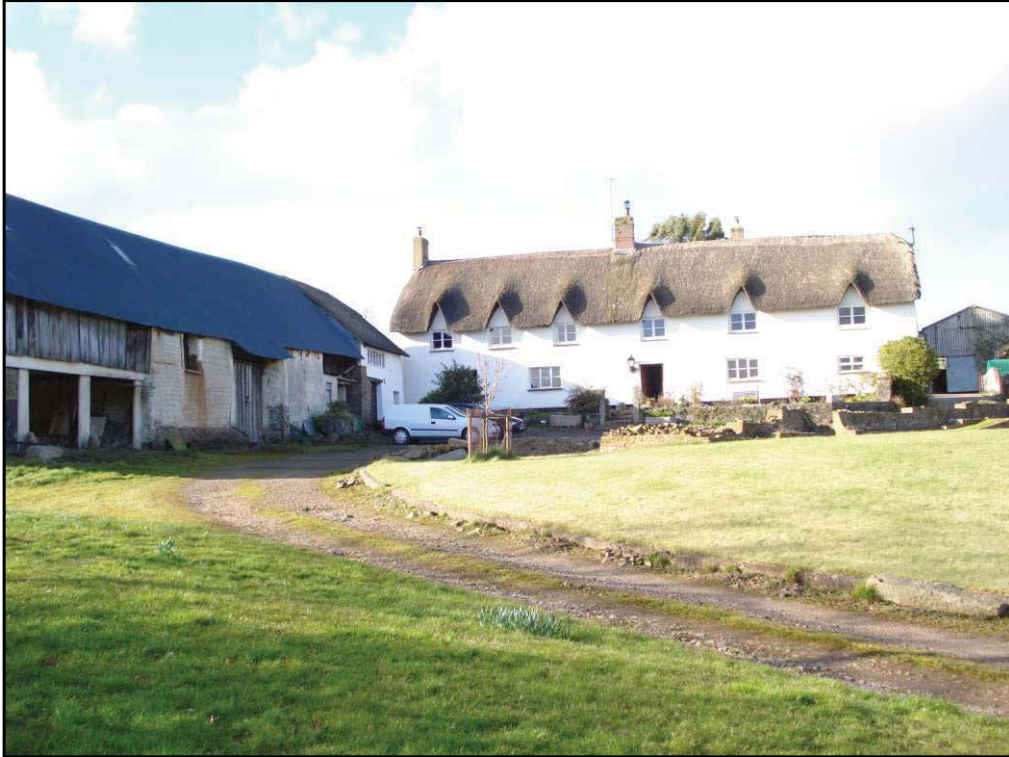
Fig. 2 General view of the buildings, looking north, showing the farmhouse with the barns lying along the western side of the former farmyard.
