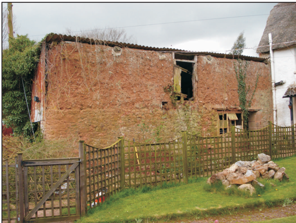
Fig. 3 General view of the north elevation of the barn.
