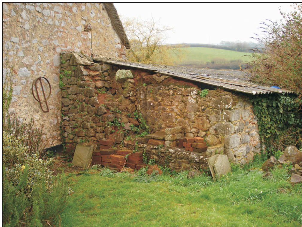
Fig.5 External view of the west wall showing the remains of the original building overlaid by 19th-century masonry relating to the rebuilding of the structure for agricultural use.
