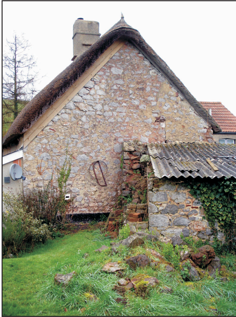
Fig. 6 View of the gable end of the cottage showing the remains of the communicating doorway in the upper parts of the gable.
