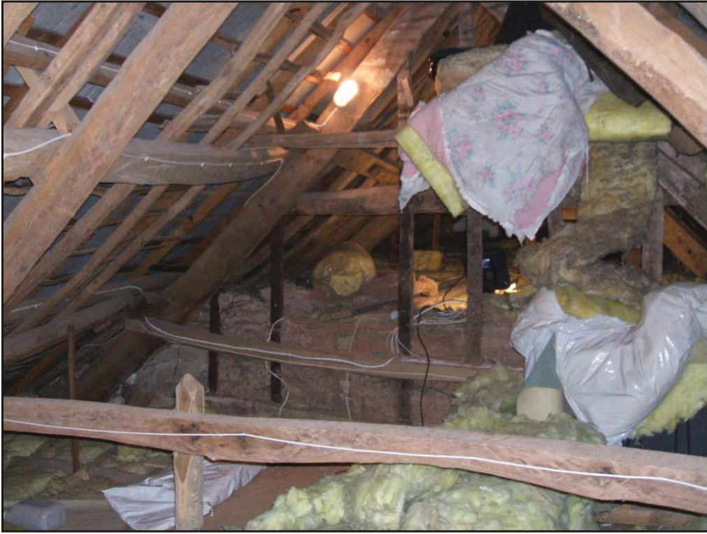
Plate 1 Roof truss 3, showing part of truss 2 in foreground, looking west.
