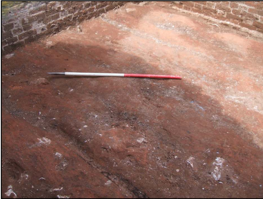
Pl. 3 Fort 1: the interior of the magazine, showing joist sockets, looking north-west. 1m scale.
