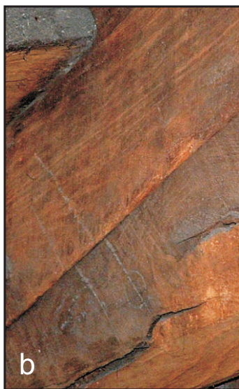
Fig. 6 Roof 1 carpentry details. (a) Projecting pegs. (b) Carpentry mark, Truss 2, NW slope. (c) Truss 2, SW slope. (d) Truss 3, SW slope.
