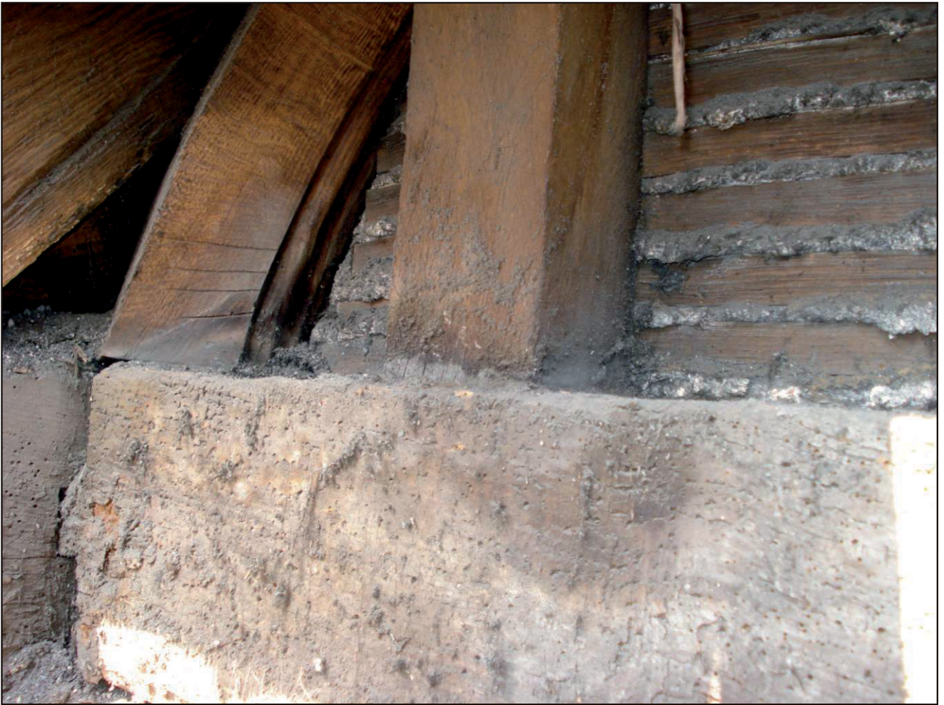
Fig. 2 Detail of the hall roof showing clean timbers and the moulded face of a windbrace protruding behind the later ceiling.
