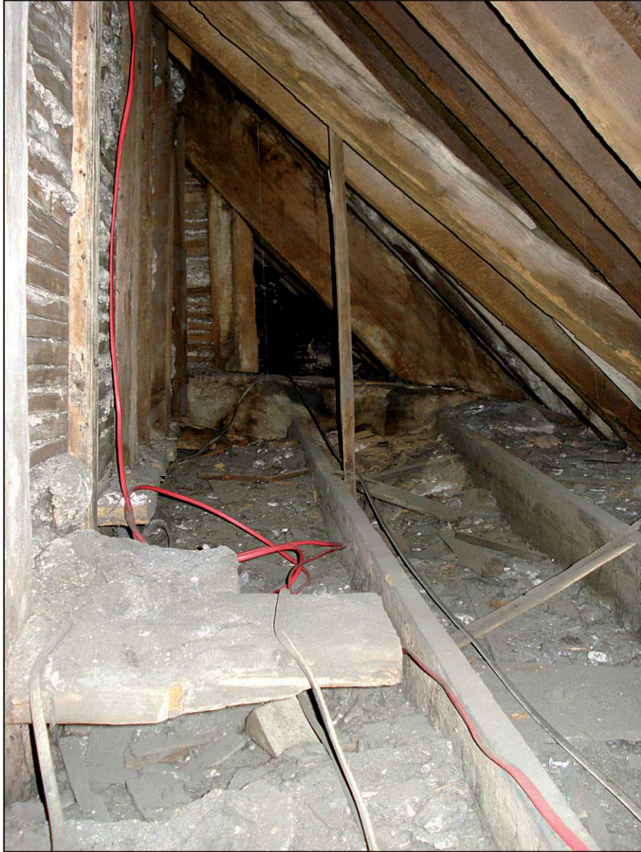
Fig. 10 Detail of the north-western foot of the truss, looking south-west.
