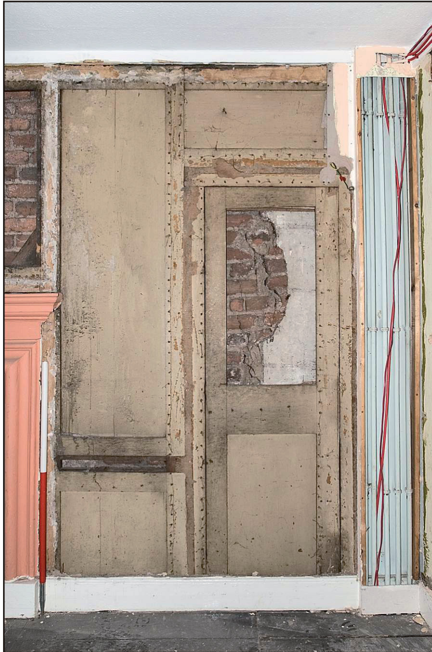
Fig. 16 Details of the panelling in the second floor, south-east room showing the anomalous door and nail marks. Scale 1m. View south.
