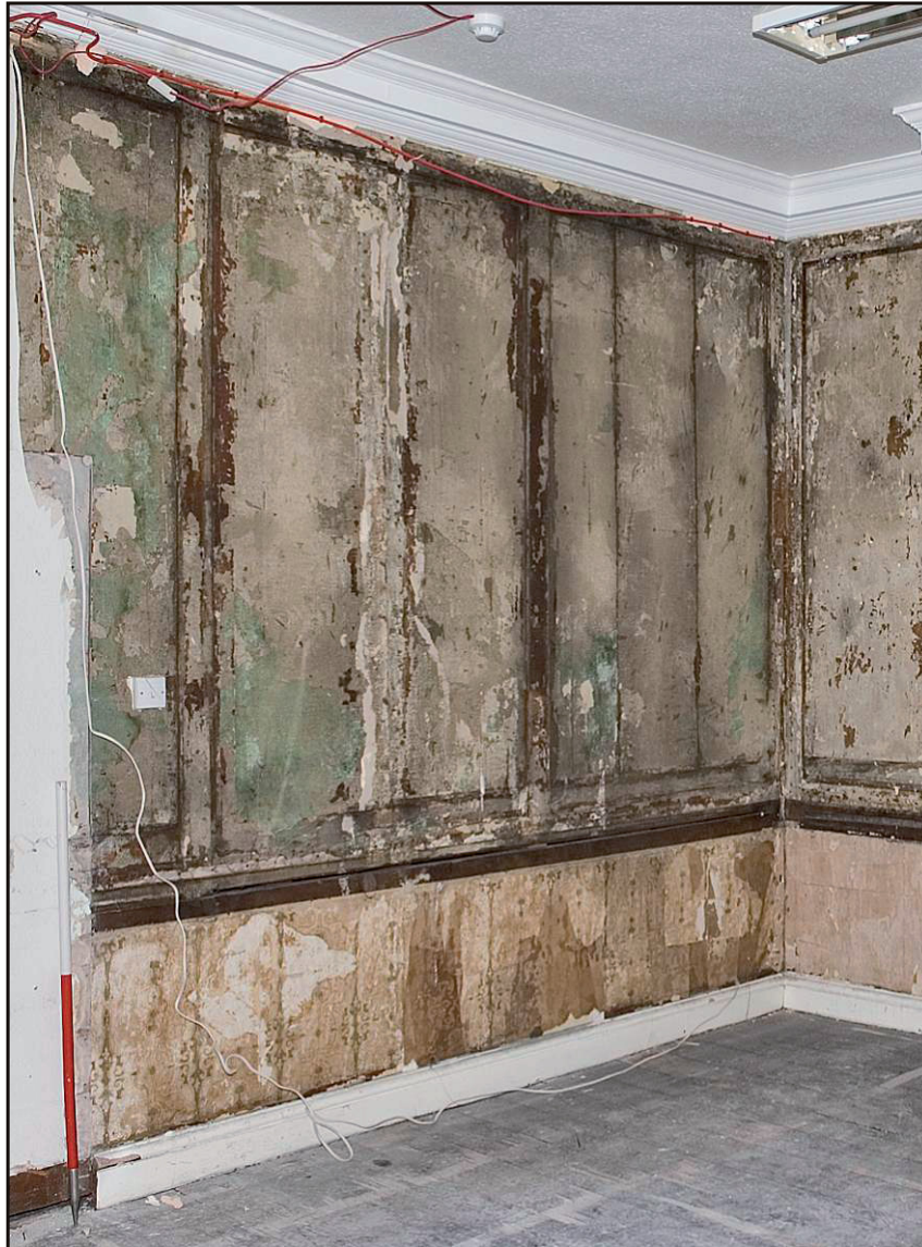
Fig. 13 View of the late 17th century bolection-moulded panelling in the ground floor west side room. Scale 1m. View south-east.
