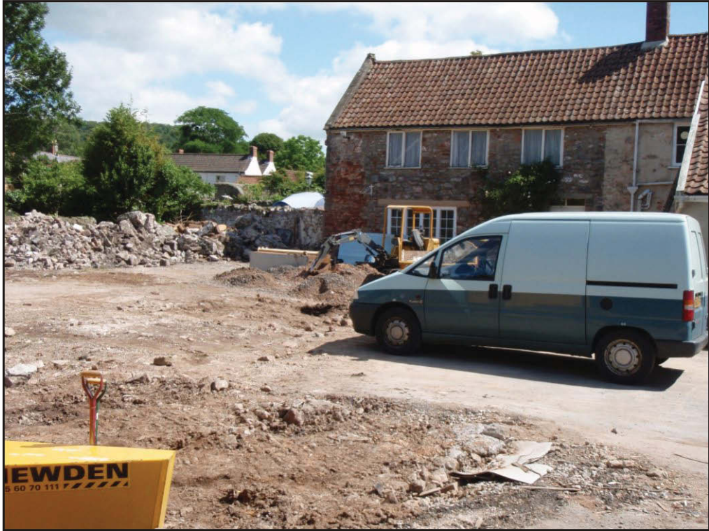
Plate 1 General site shot before excavation. Looking east.
