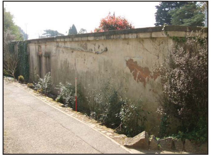
Plate 2 The north elevation of the Report and Control Center showing the post-war extension, looking southeast. 1m scale.
