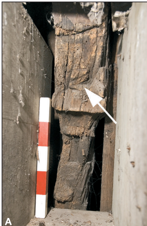
Pl. 8 Details of the first-floor corner jetty brackets showing similar remains of carving detail possibly depicting draped clothing. (A) east-end jetty post. (B) west-end jetty post. Scale 0.25m. View south-east.
