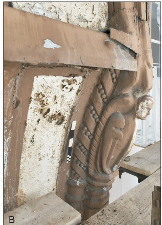
Pl. 2 Second-floor corner jetty post figures, (A) C18th/19th cast gypsum angel at the east end, (B) C20th cast cement angel and adjacent spiral ribbon and bead-moulded jetty bracket at the west end. Scale 0.25m. Views (A) south-east, (B) south-west.
