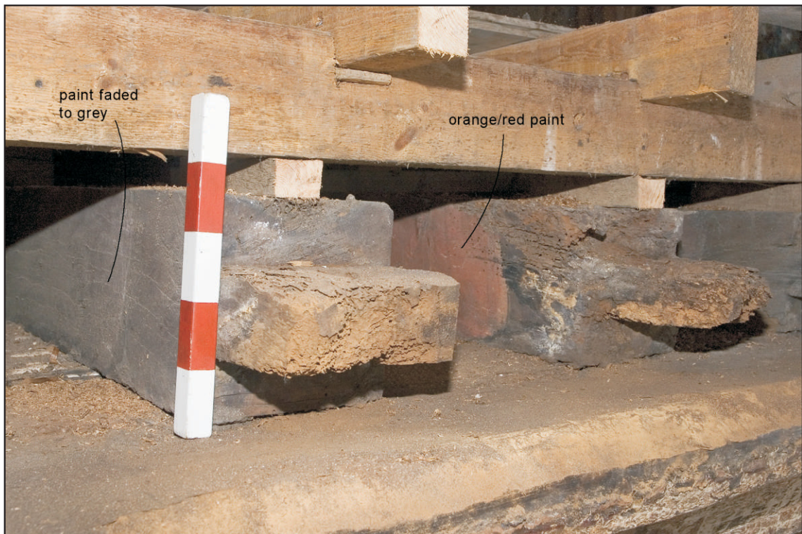
Pl. 17 View of the second-floor joists, after removal of the girding beam, showing alternate colours painted onto both sides and also presumably the soffits. Scale 0.25m. View south.
