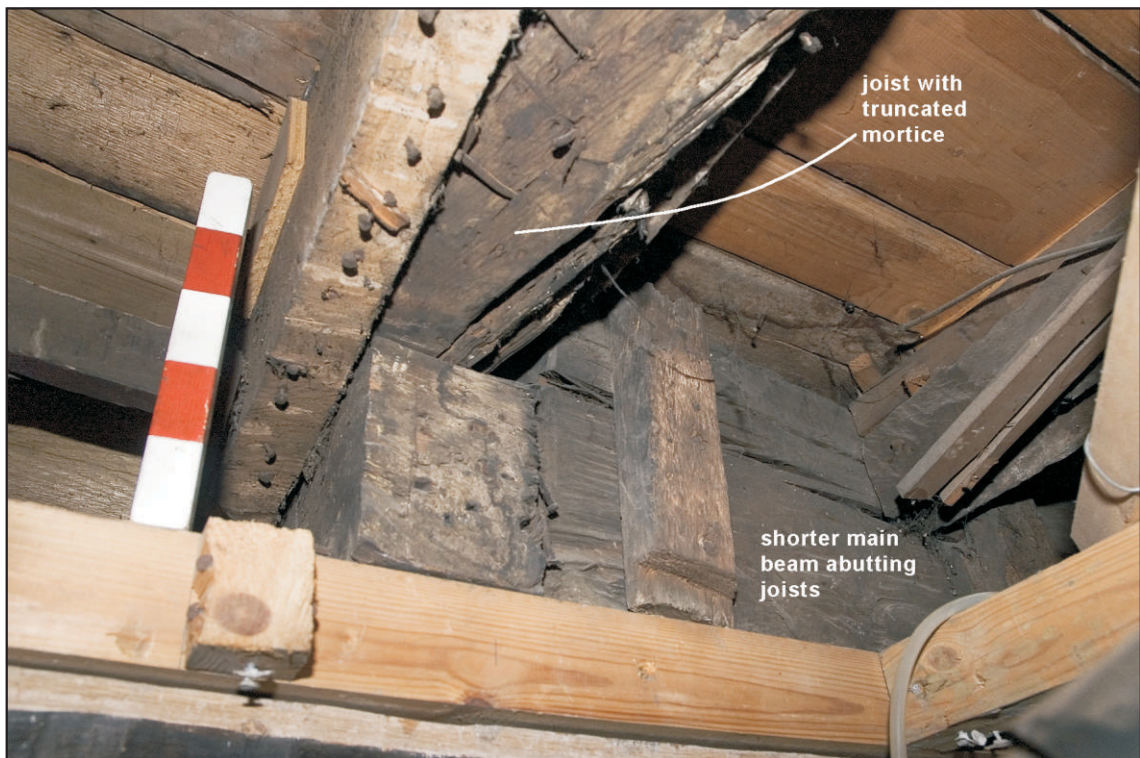
Pl. 23 View of the shorter main beam in the third bay of the ground-floor ceiling of the north-west room showing the abutment of its south-east end against the joists marking the former position of a passage screen. Scale 0.25m. View south.
