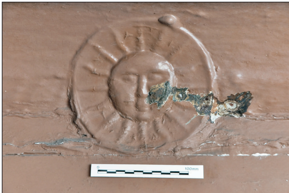
Pl. 10 Detail of the C18th/early C19th fire insurance plaque attached to the first-floor covered window head. The sun emblem appears to be pressed in tin-plated iron. Scale 100mm. View south-east.
