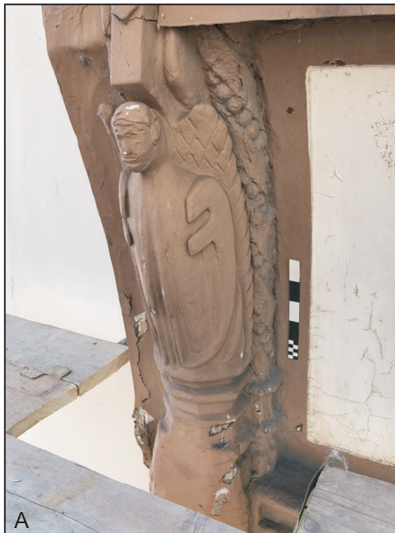
Pl. 2 Second-floor corner jetty post figures, (A) C18th/19th cast gypsum angel at the east end, (B) C20th cast cement angel and adjacent spiral ribbon and bead-moulded jetty bracket at the west end. Scale 0.25m. Views (A) south-east, (B) south-west.
