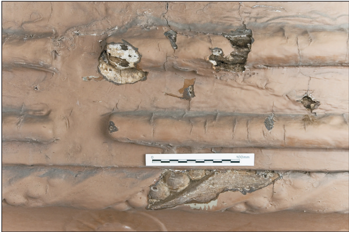
Pl. 3 Detail of the roll-moulded girthing beam with spiral ribbon and bead moulding below. Note thickness of paint layers obscuring the carving detail. Scale 100mm. View south-east.
