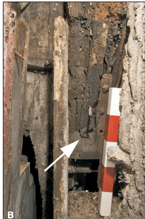
Pl. 8 Details of the first-floor corner jetty brackets showing similar remains of carving detail possibly depicting draped clothing. (A) east-end jetty post. (B) west-end jetty post. Scale 0.25m. View south-east.
