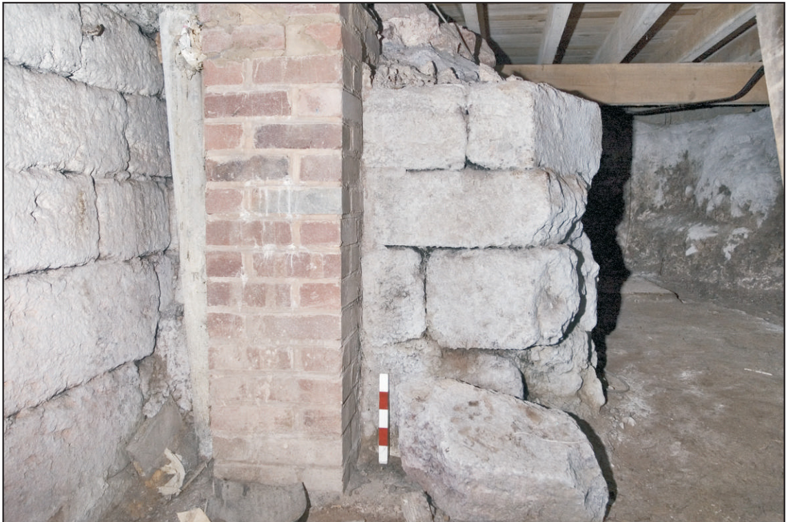
Pl. 19 View of the stump of the breached south-eastern cellar wall showing the splayed reveal of a former window. Scale 0.25m. View south-east.
