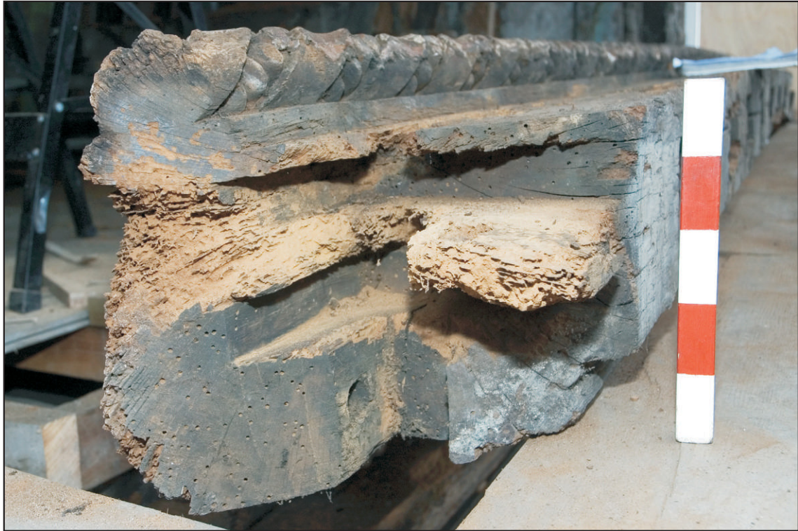
Pl. 14 Detail of the second-floor moulded girding beam after removal from the facade showing the mitred joint incorporating three interwoven tenons. Note the mortice with peg hole for the upper corner post. Beam is viewed upside down. Scale 0.25m.
