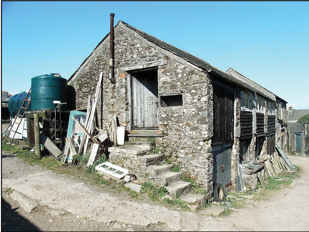
Plate 5 The linhay, west and south elevations. View to northeast.
