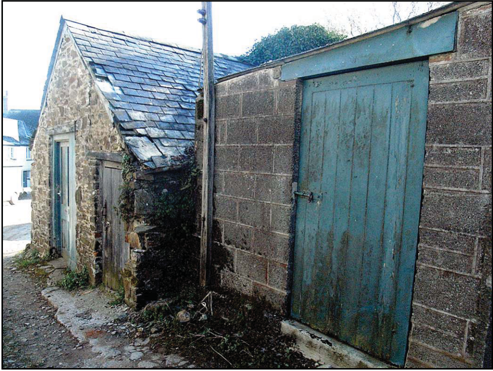
Plate 7 The office and wood shed, northwest elevation. View to east.
