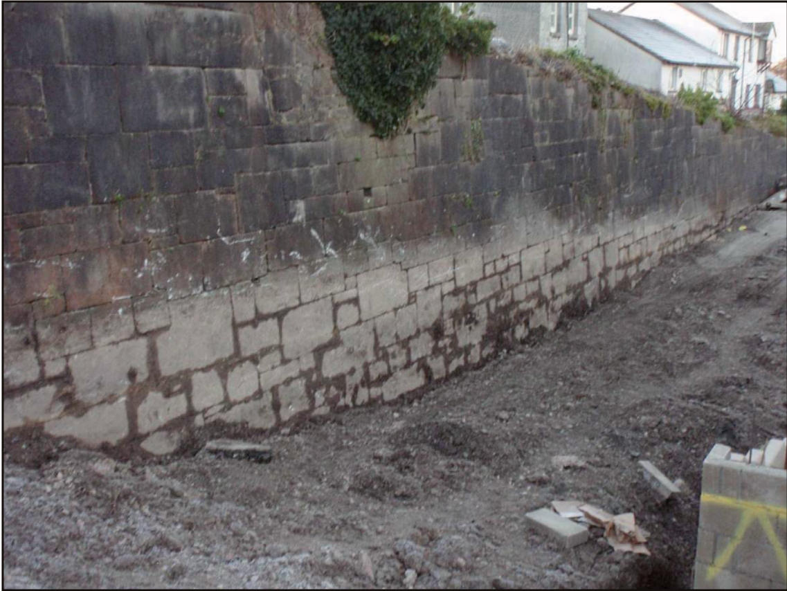
Photo 1 The scarp wall (of Marlborough Bastion), looking southwest.
