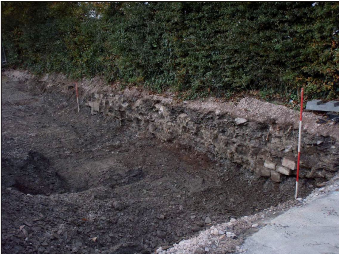
Photo 2 The remains of the counterscarp wall, looking northwest. 1m and 2m scales.
