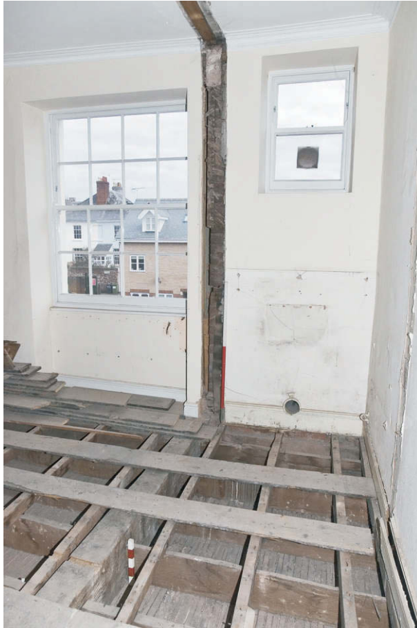
Photo 10. The second-floor rear room following the removal of a modern partition and the raising of boards, exposing a large floor beam and the original window splay in the rear wall. Scale 0.25m. View north-east.
