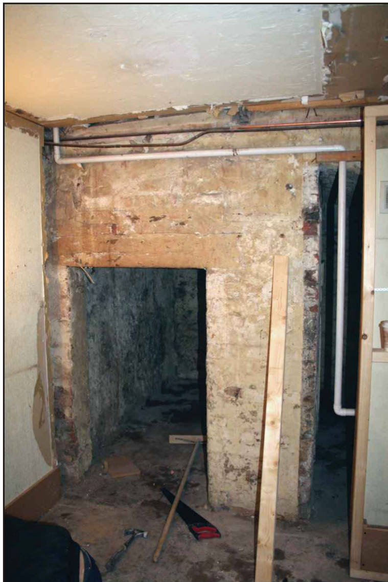
Photo. 2 The low door in the cellar in the basement, looking northwest.
