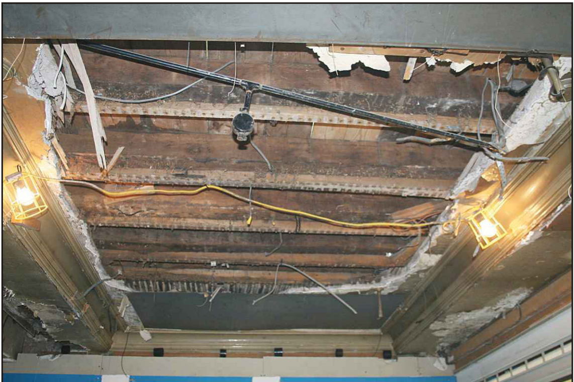
Photo. 4 The ground-floor ceiling showing two phases of joists and the wooden cornice, looking northeast.
