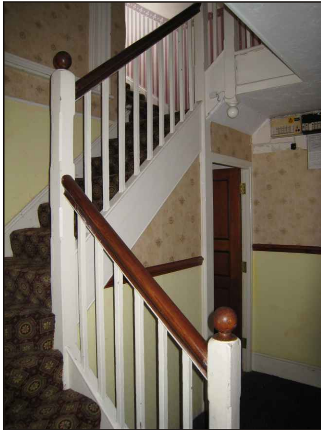
Photo. 5 The servants' stairs to the first floor photographed in 2007, looking southwest (Kathy Metcalfe, Exeter City Council).
