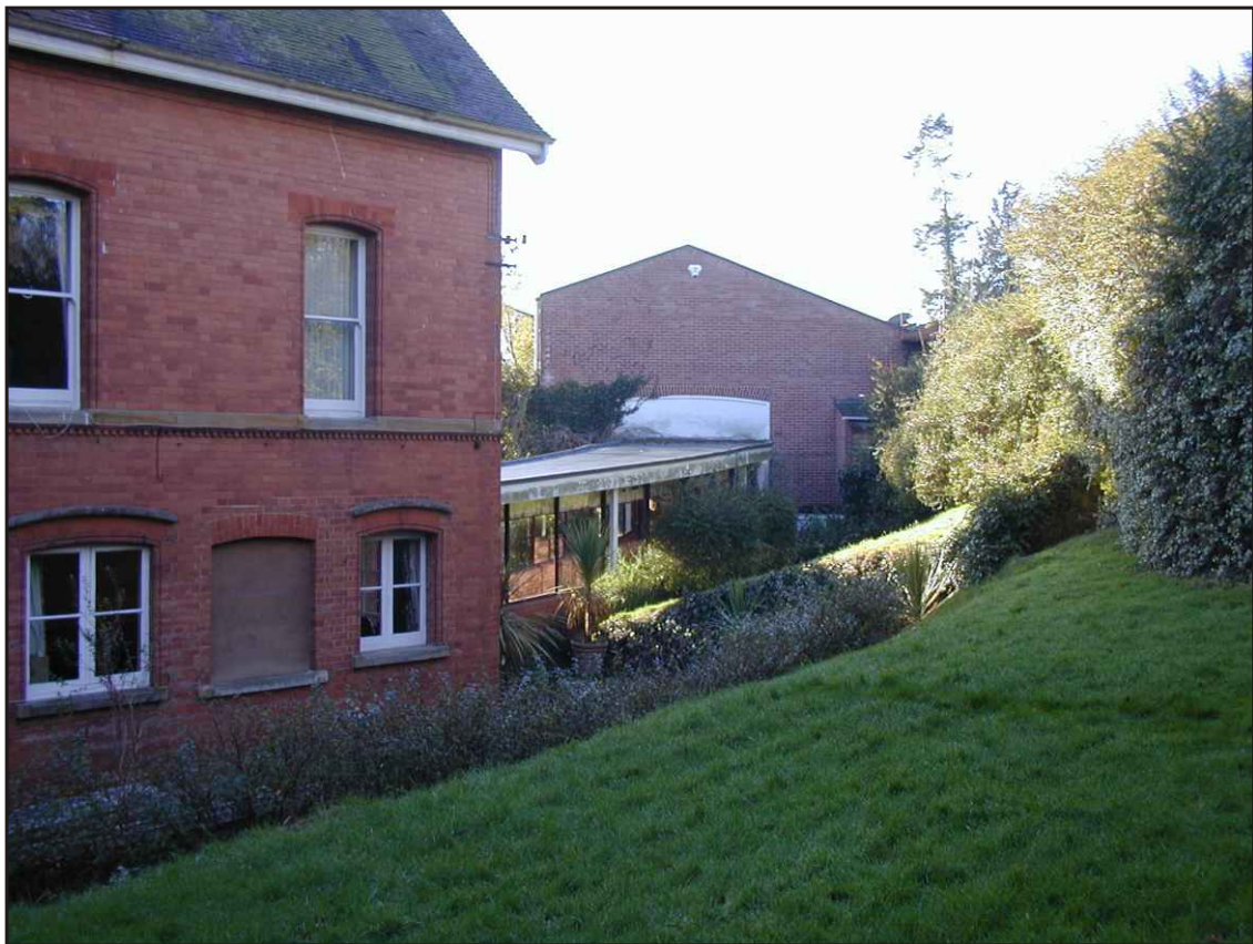
Photo. 8 The north elevation photographed in 2005 showing C20 replacement window openings and link to the dining hall, looking west (Exeter Archaeology).
