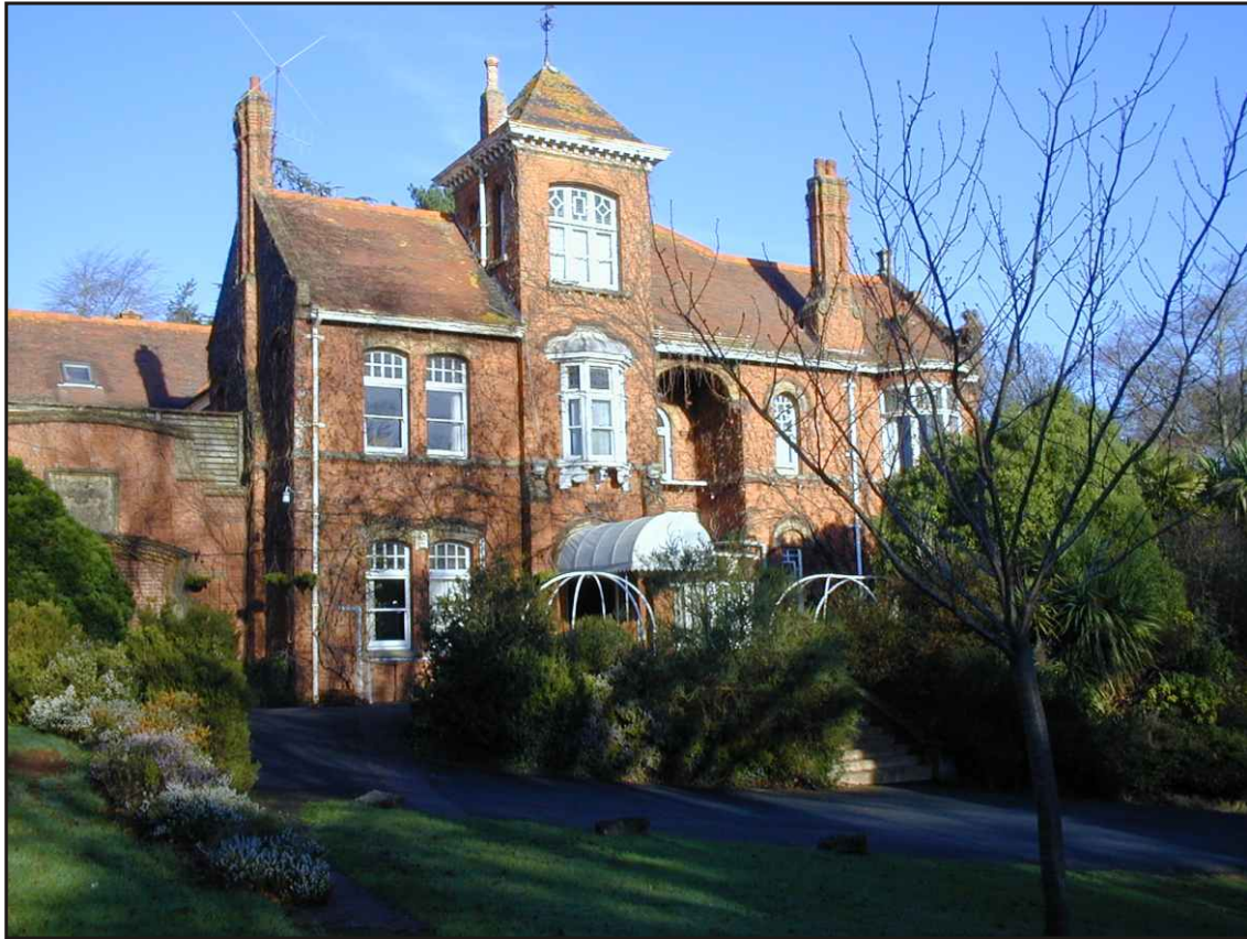
Photo. 1 The south elevation photographed in 2005, looking north (Exeter Archaeology).
