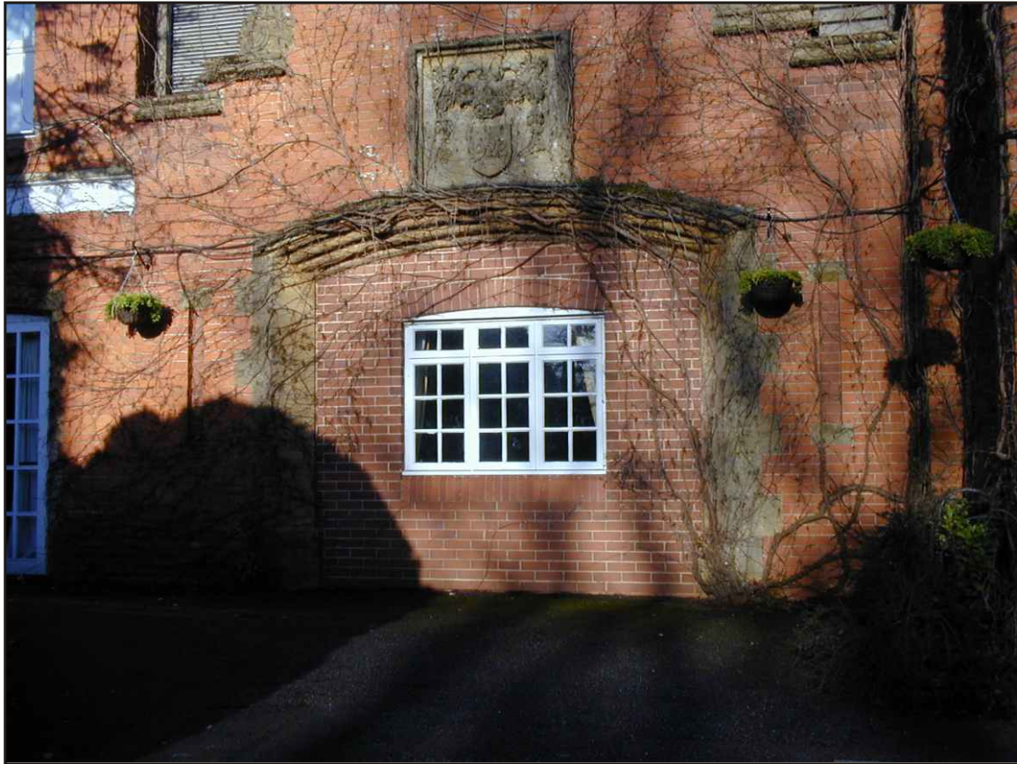
Photo. 7 The blocked carriage entrance in the 1922 wall enclosing the courtyard photographed in 2005, looking northwest (Exeter Archaeology).
