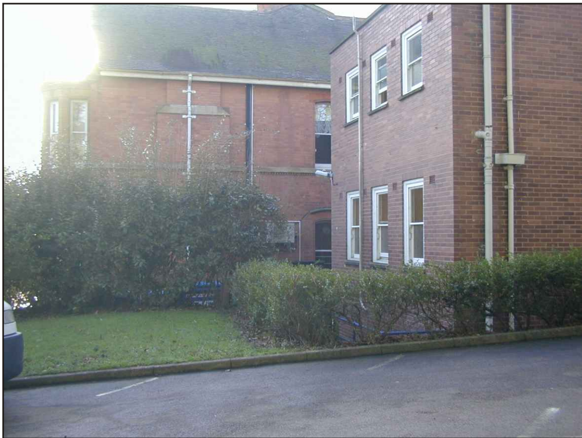
Photo. 2 The north elevation photographed in 2005 showing late C20 extension, looking south (Exeter Archaeology).
