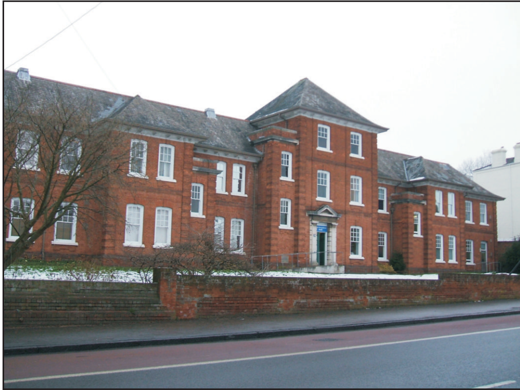
Plate 1 The former Children's Home, showing two phases of low brick wall alongside Heavitree Road. Looking north-east.
