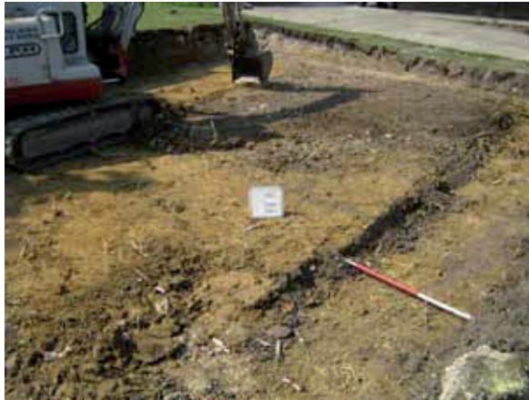
Garage area, looking north-west
