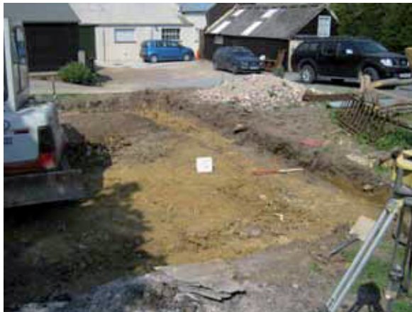
Garage area, looking north-east
