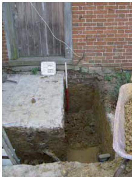
Porch area, looking west
