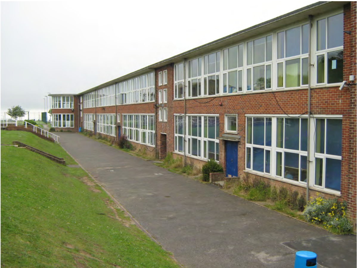
Fig. 19 - View of rear of main block facing South
