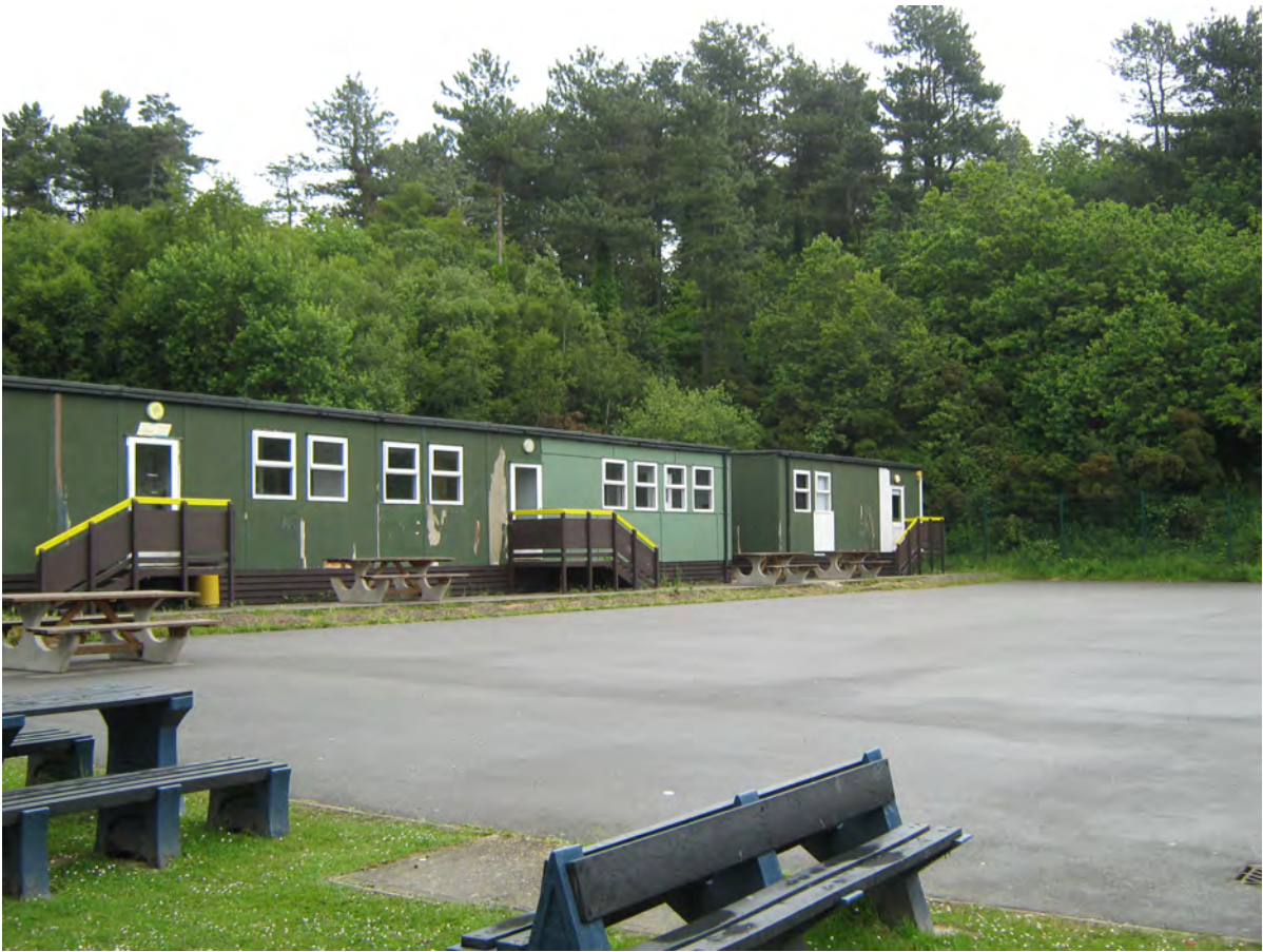
Fig. 16 - View of temporary blocks facing North East
