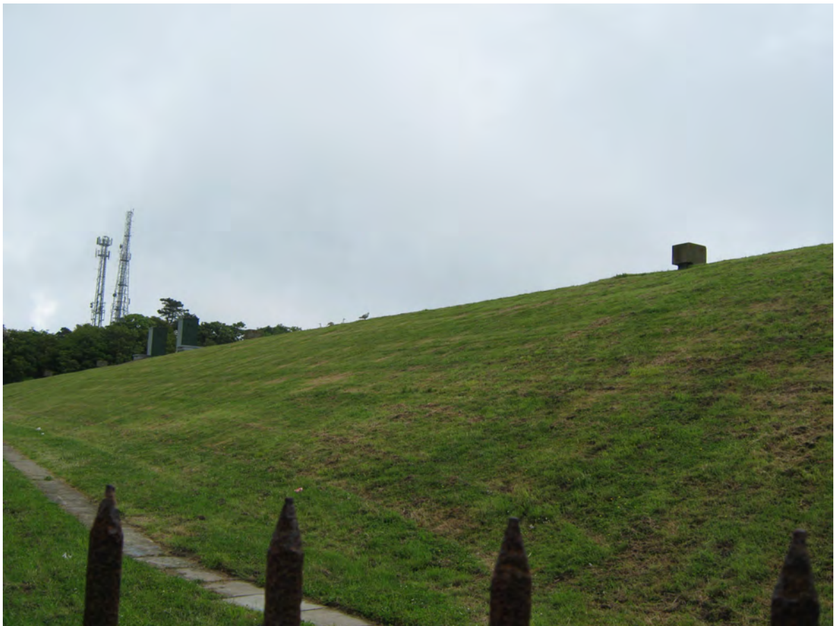
Fig. 22 - View of covered reservoir facing North East
