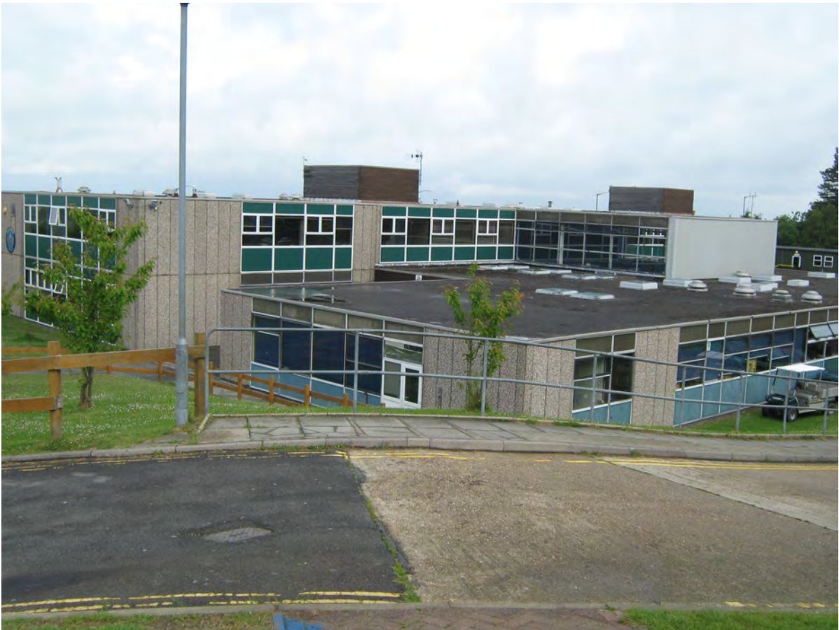
Fig. 17 - View of A block facing North West
