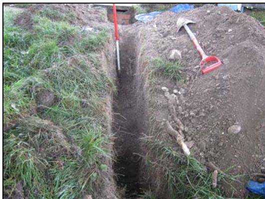
Pipe trench south of walls
