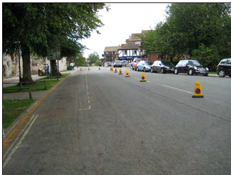
Plate 1: South-westward view along the active roadway
