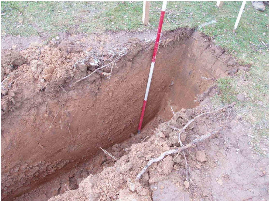
Fig. 3.2: Footing for new dwelling, looking west
