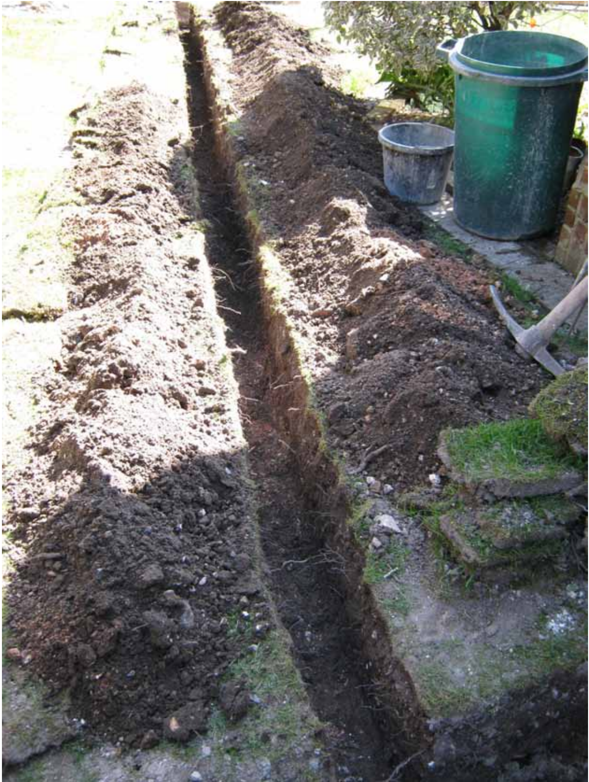
Pipe trench looking east
