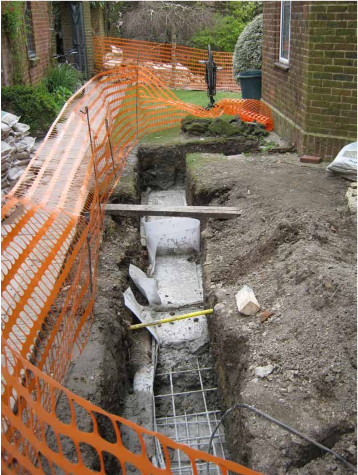
Extension footings looking north-east
