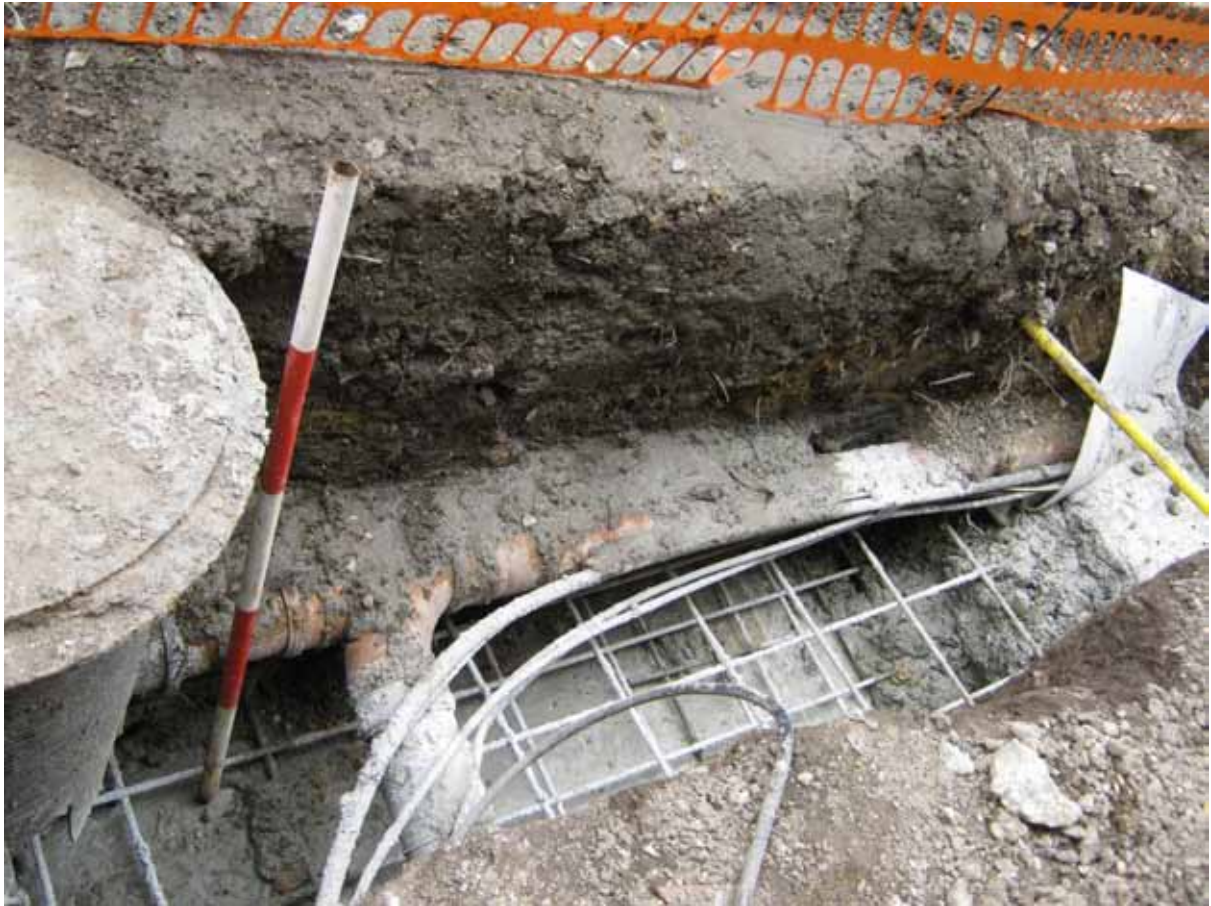
Footing trench looking north
