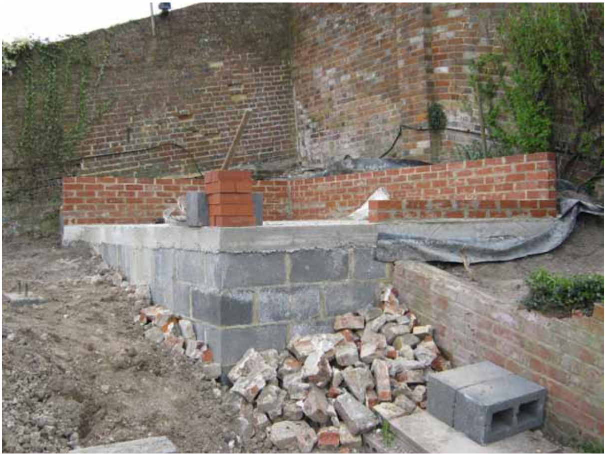
Summer House foundations looking west, note town wall and inner bank
