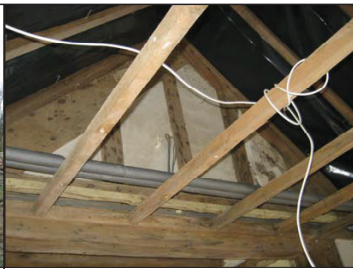
Fig. 2.2: Original S extent of building at SW corner
