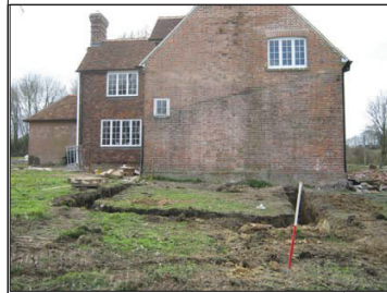
Fig. 2.1: Trenching for garden room
