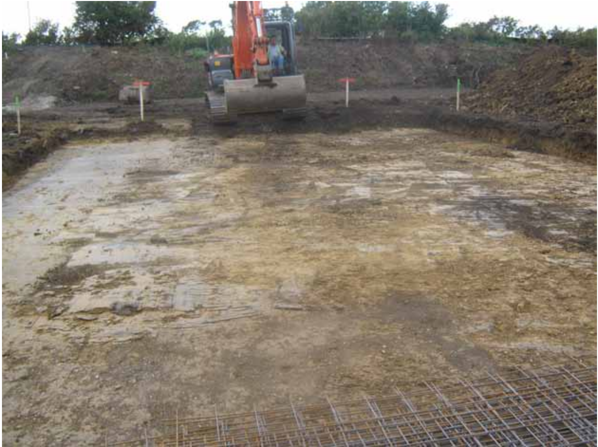
Plate 2: Hoeford ground reduction viewed from the east
