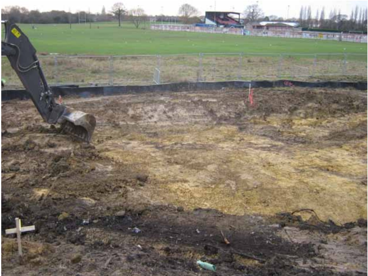
Plate 1: Redlands Lane ground reduction viewed from the north-east
