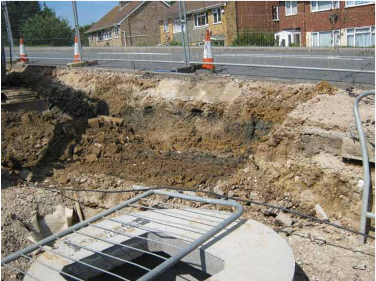
Plate 4: Manhole at Tichborne Way, viewed from the east
