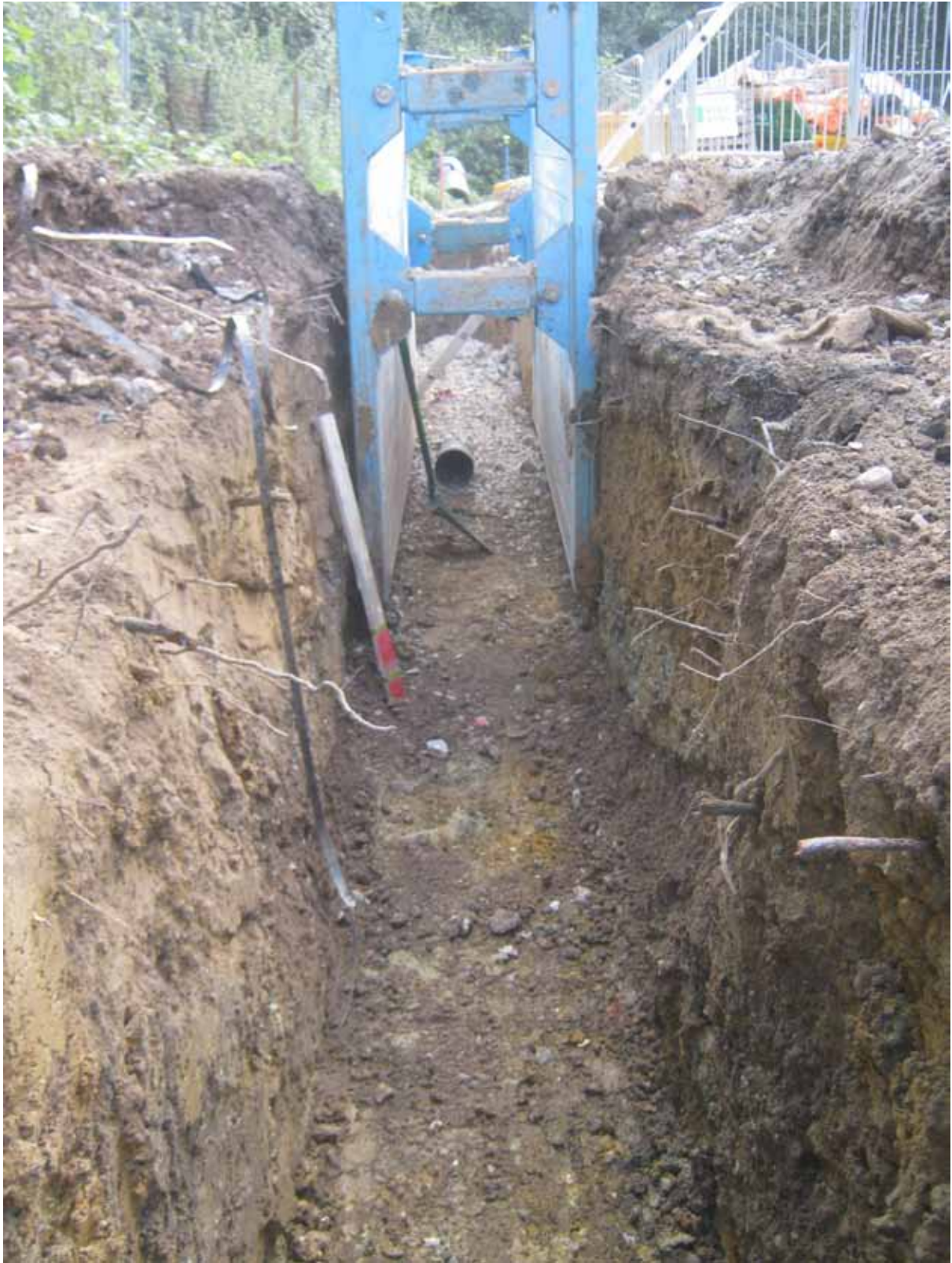
Plate 5: Tichborne Way trenching viewed from the south
