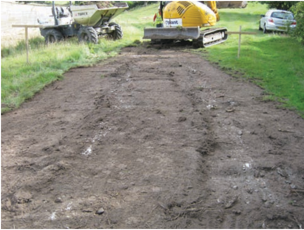
Topsoil strip for Haul Road with consolidated wheel ruts evident
