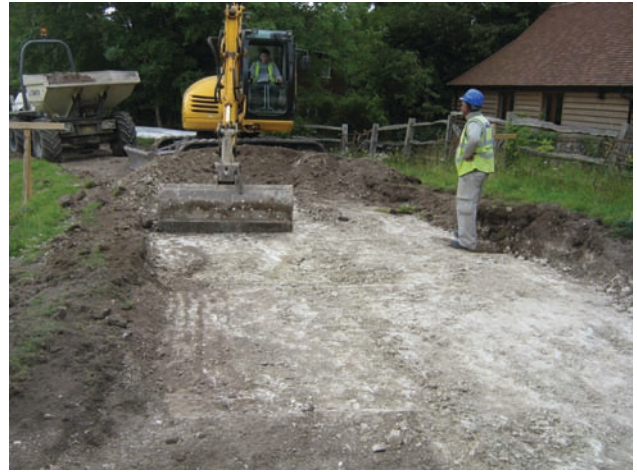
Machine reduction of road strip
