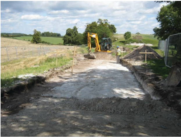
Machine reduction of road strip
