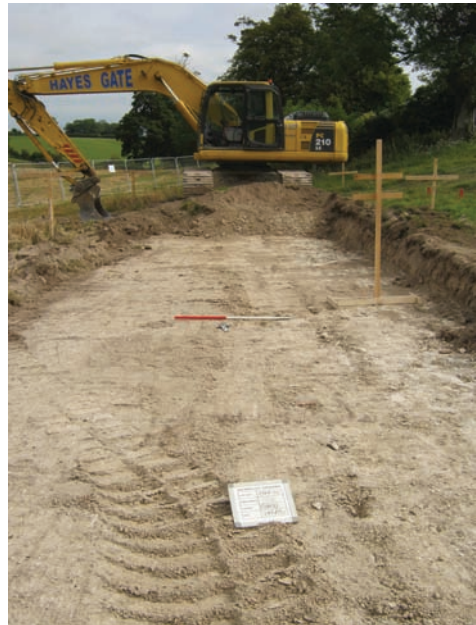
Machine reduction of road strip
