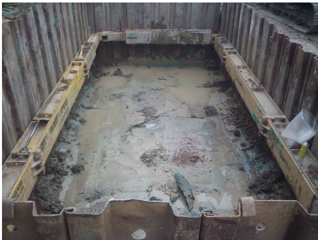
Lower level of Reed Bed excavation
