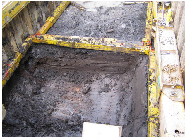
Section 3 during excavation
