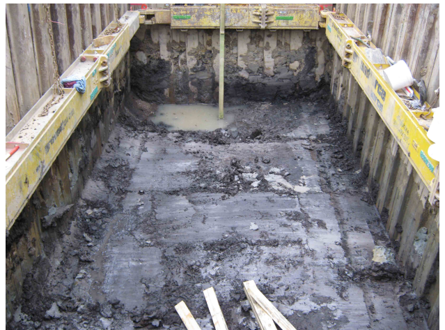
Maximum extent of Reed Bed excavation showing organic alluvium 012
