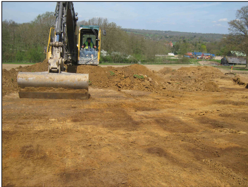
South field during stripping of topsoil
