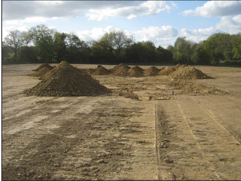
North field after stripping of topsoil and colluvium
