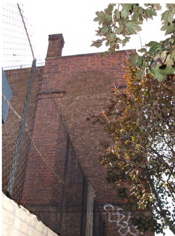
Plate 25: Phase 2 – Block 2a, the east end elevation
