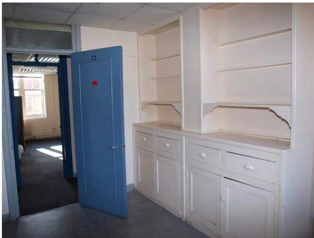
Plate 40: Phase 2 – Block 2a, room S5 on the second floor, with built in dresser
