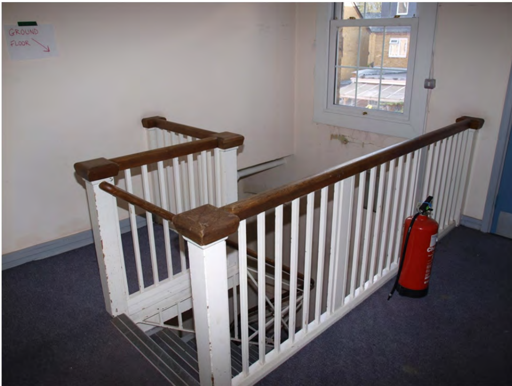
Plate 19: Phase 1 – Block 1c staircase, first floor detail
