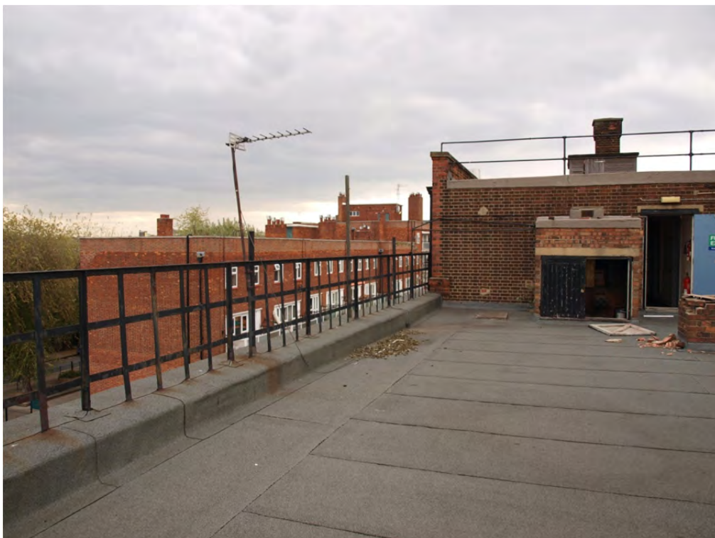
Plate 30: Block 2a roof – east end, with small structure built to house flue/extractor
