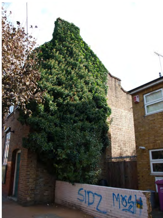
Plate 49: Block 3 – west end wall detail
