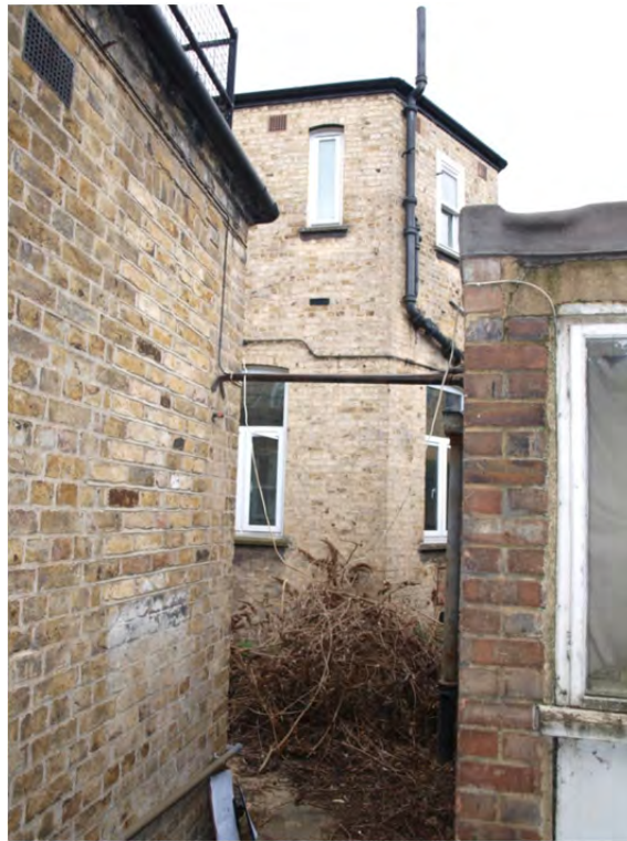
Plate 5: Phase 1 or just after, the west facing elevation of Block 1d
