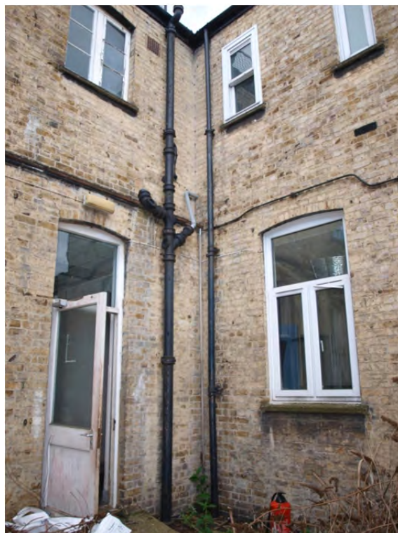
Plate 4: Phase 1 – west and north facing elevations of Blocks 1c and 1e
