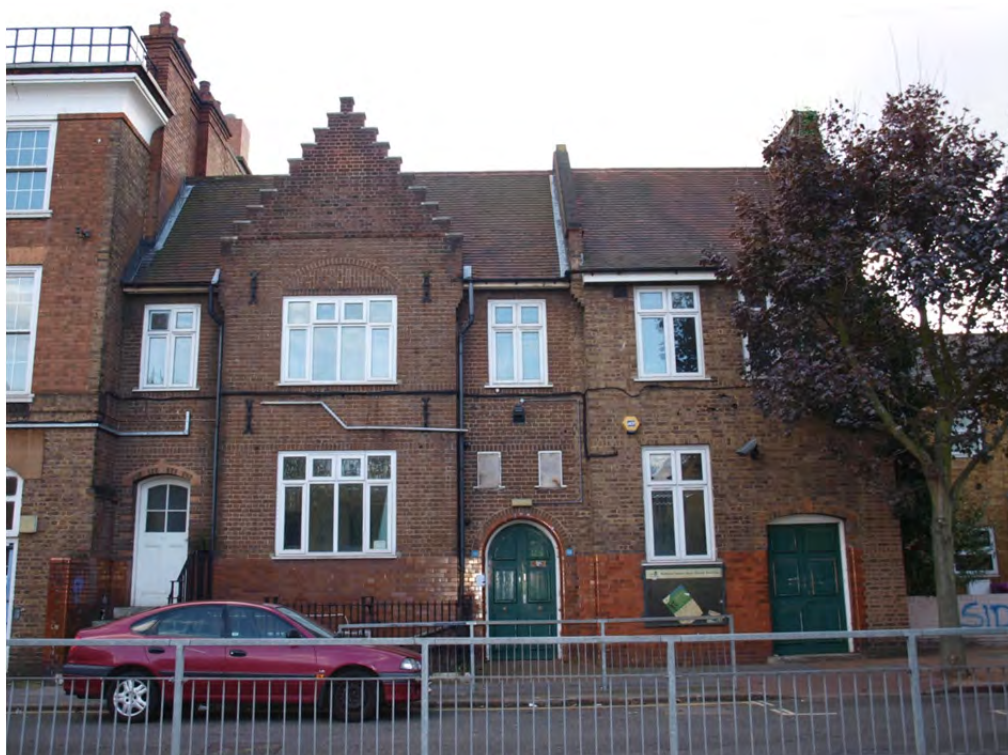
Plate 48: Phase 1 and possibly 2, the Block 3 addition stitched into the Phase 1 range, designed to match the existing Block 1a principal elevation details
