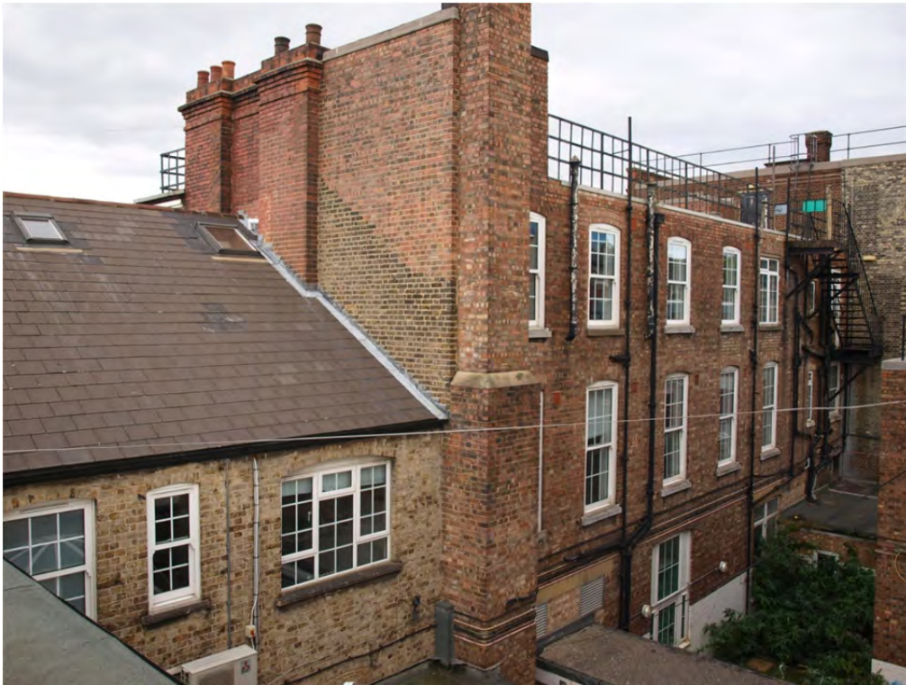
Plate 3: Phase 1 and 2 – rear elevations of Blocks 1a and 2a
