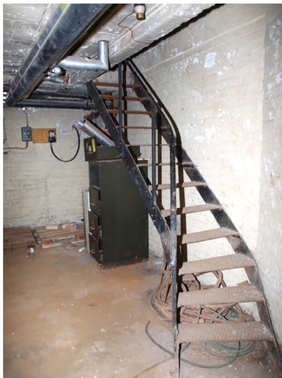
Plate 36: Phase 2 – Block 2a, the cellar below the east tower (B3)
