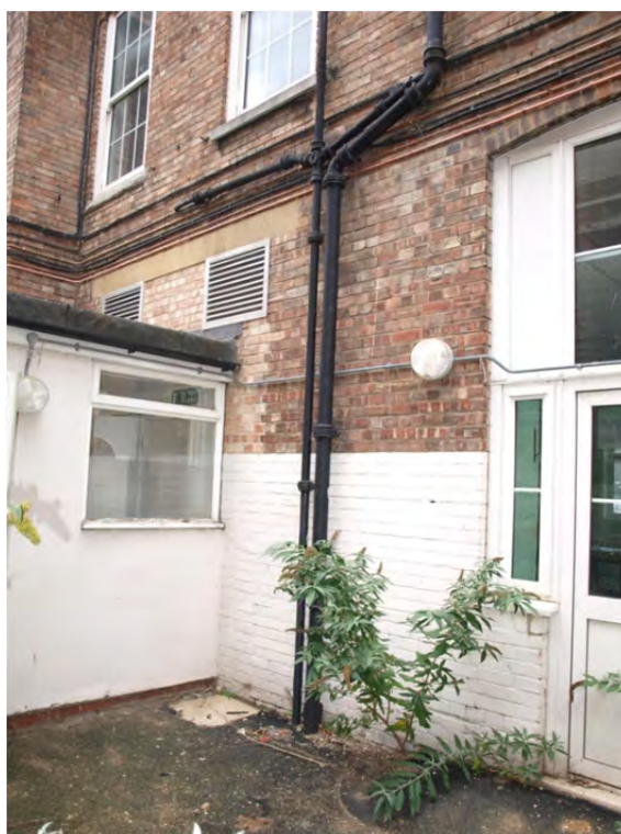
Plate 26: Phase 2 with modifications, part of the south side of Block 2a, with the late 20th century link addition (Block 7)
