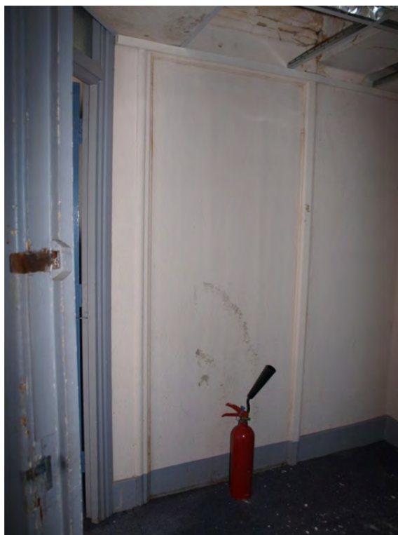
Plate 46: Phase 2 – Block 2b, the in-filled former second floor entrance to the east arm lift
