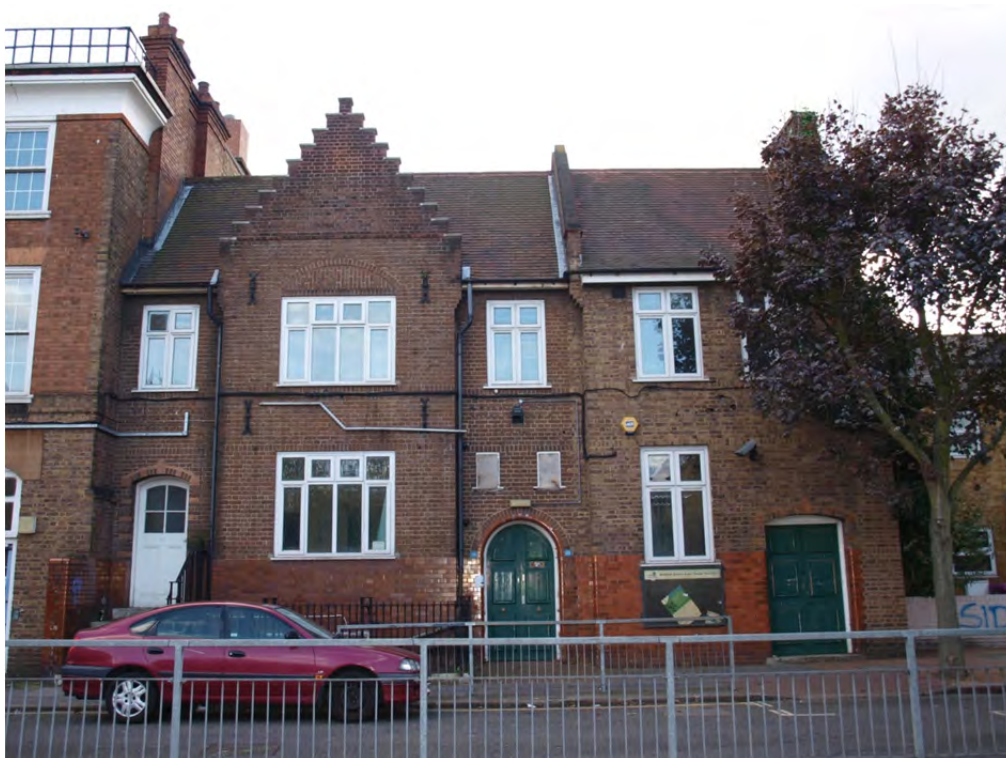
Plate 2: Phase 1 and 2 – the principal (Underwood Rd) elevation of Blocks 1a and 3, (2a just visible)
