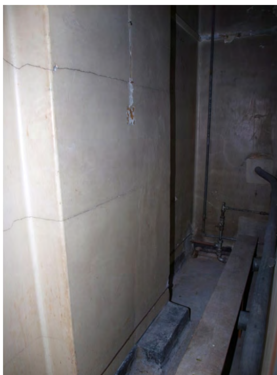
Plate 42: Block 2a – second floor, former chimney breast, now within small room created when WC facilities were added to the west, to house pipes
