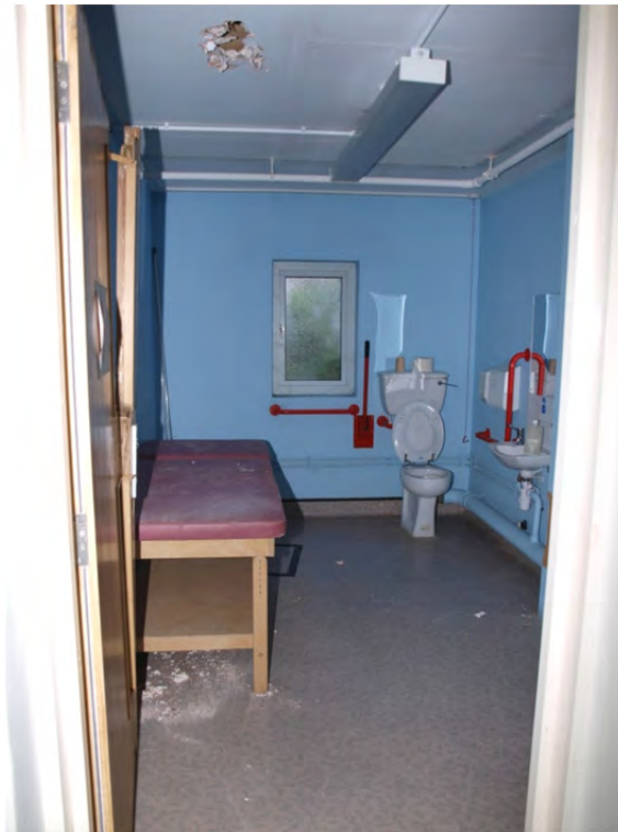
Plate 37: Phase 4 – Block 8, interior of the north room (G50)
