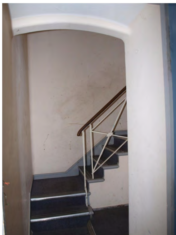
Plate 18: Phase 1 – Block 1c staircase, ground floor detail
