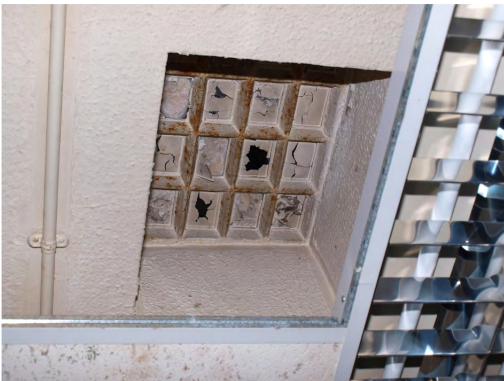
Plate 20: Phase 1 – Block 1e, first floor room F28, detail of former roof-light:
