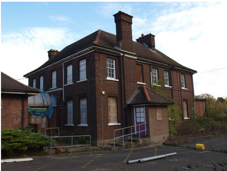
Building 1 from the south-west
