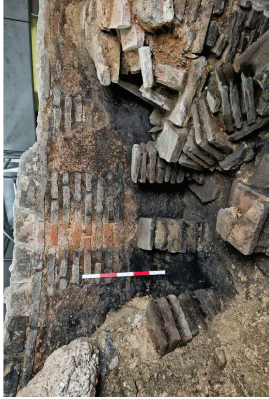
Shot of internal elevation of apse (section 1)
