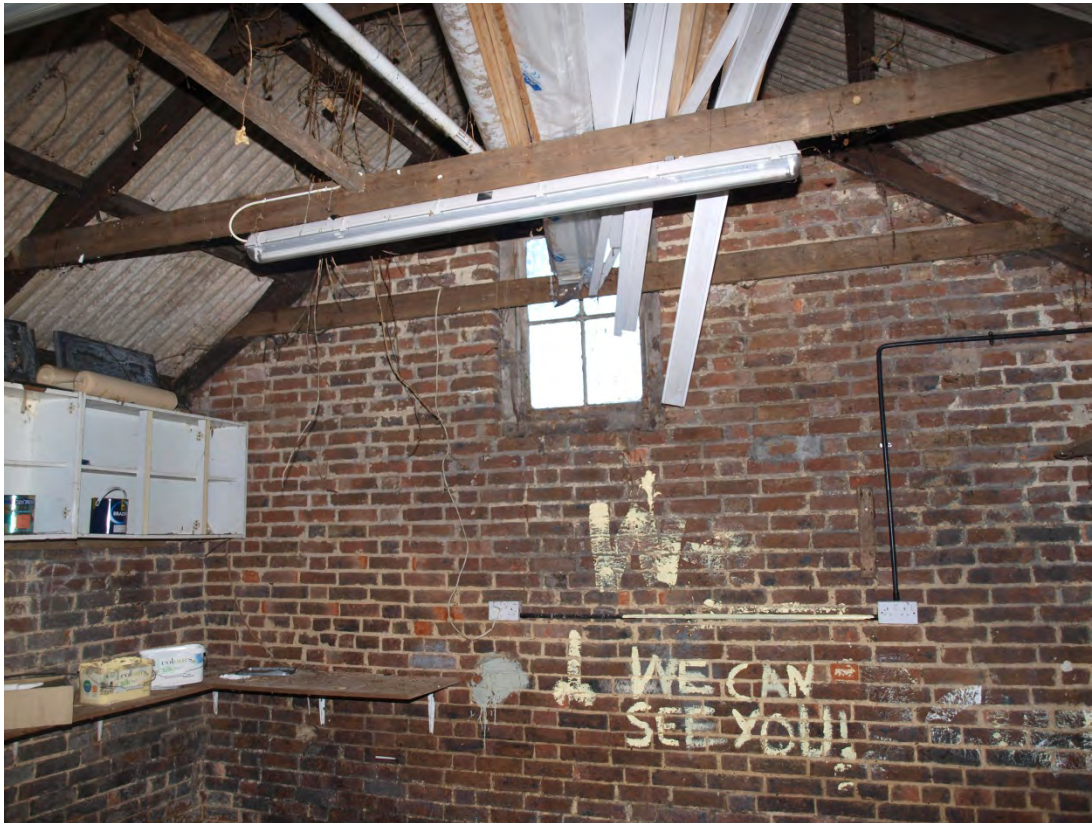
Plate 23: View of the interior of the outbuilding, looking north-west (14)
