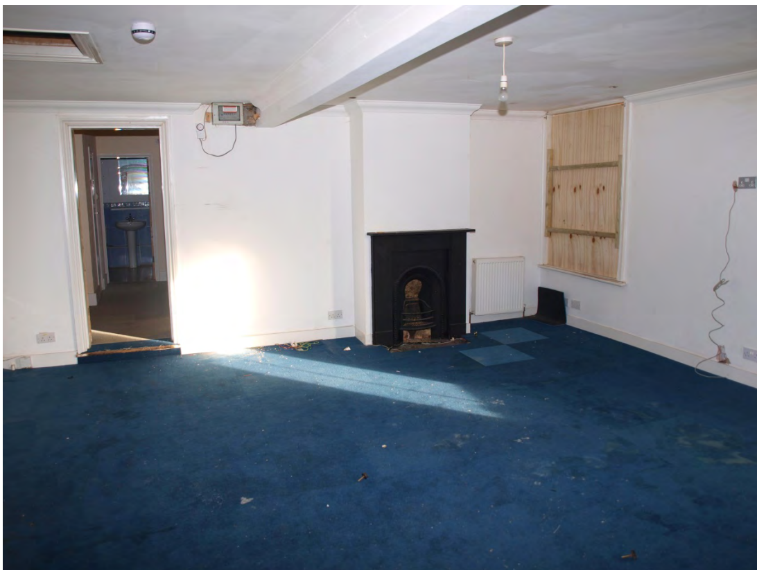
Plate 18: Large room within southern end of principal range, looking north (18)
