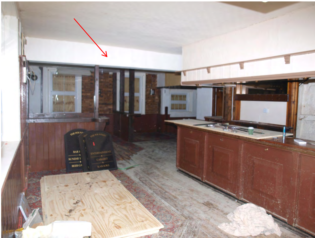
Plate 5: Main bar area within southern end of principal range, looking south. Line of original partition wall highlighted (18)
