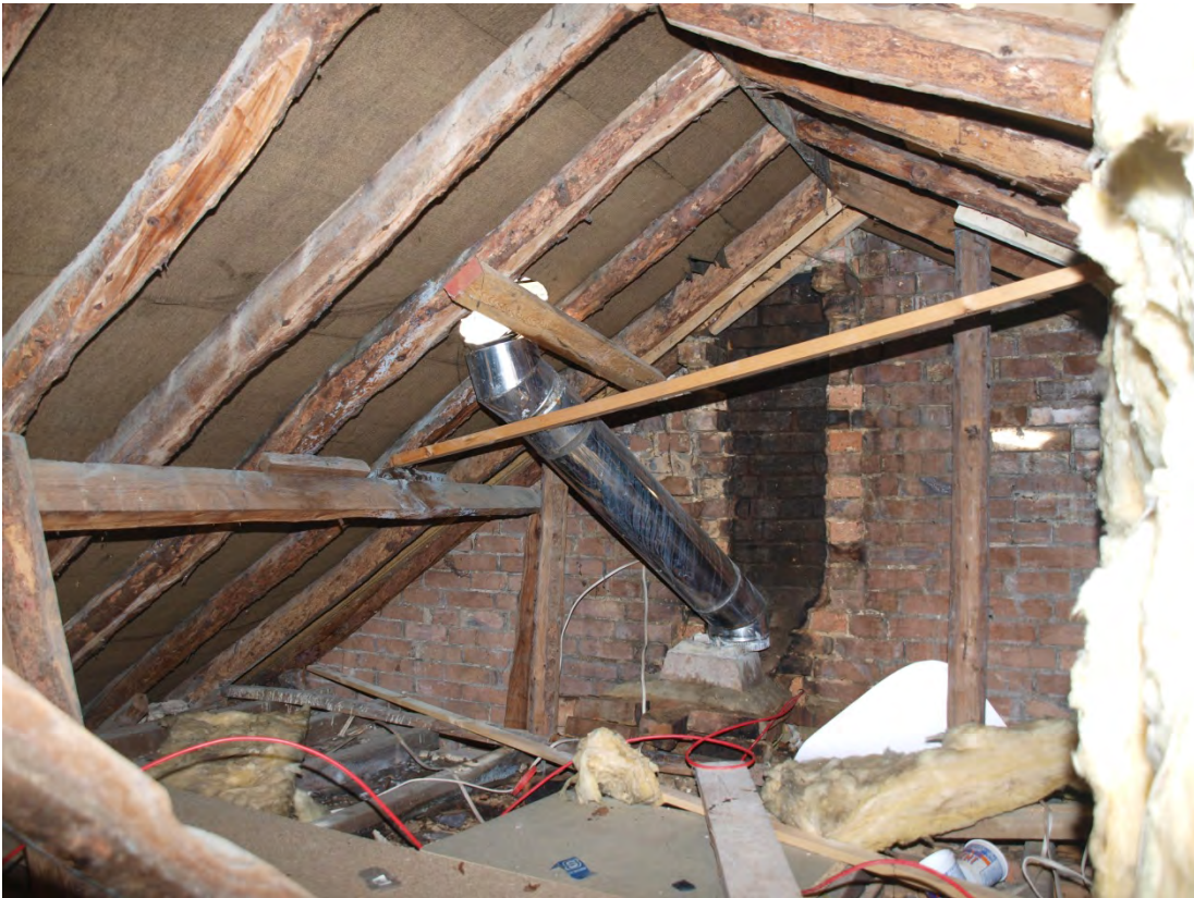
Plate 21: Roof over 19 th century rear addition, looking south-west (38)
