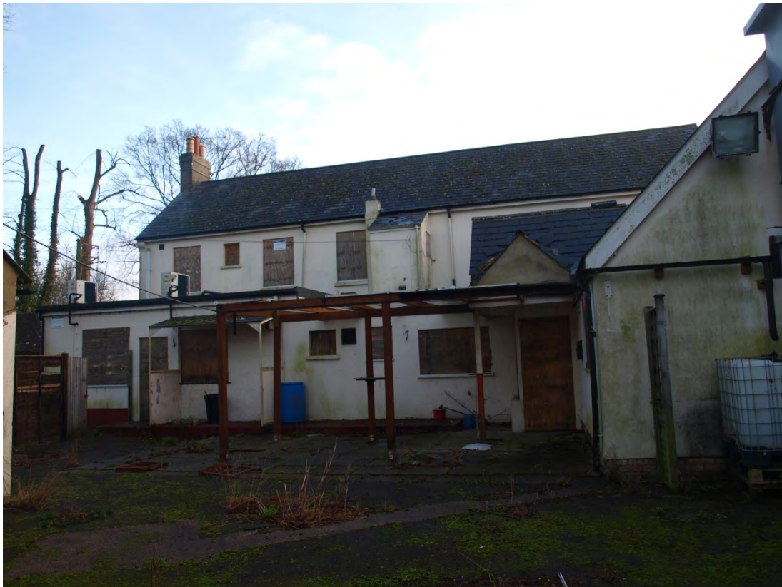
Plate 4: Rear (west) elevation, looking east (8)
