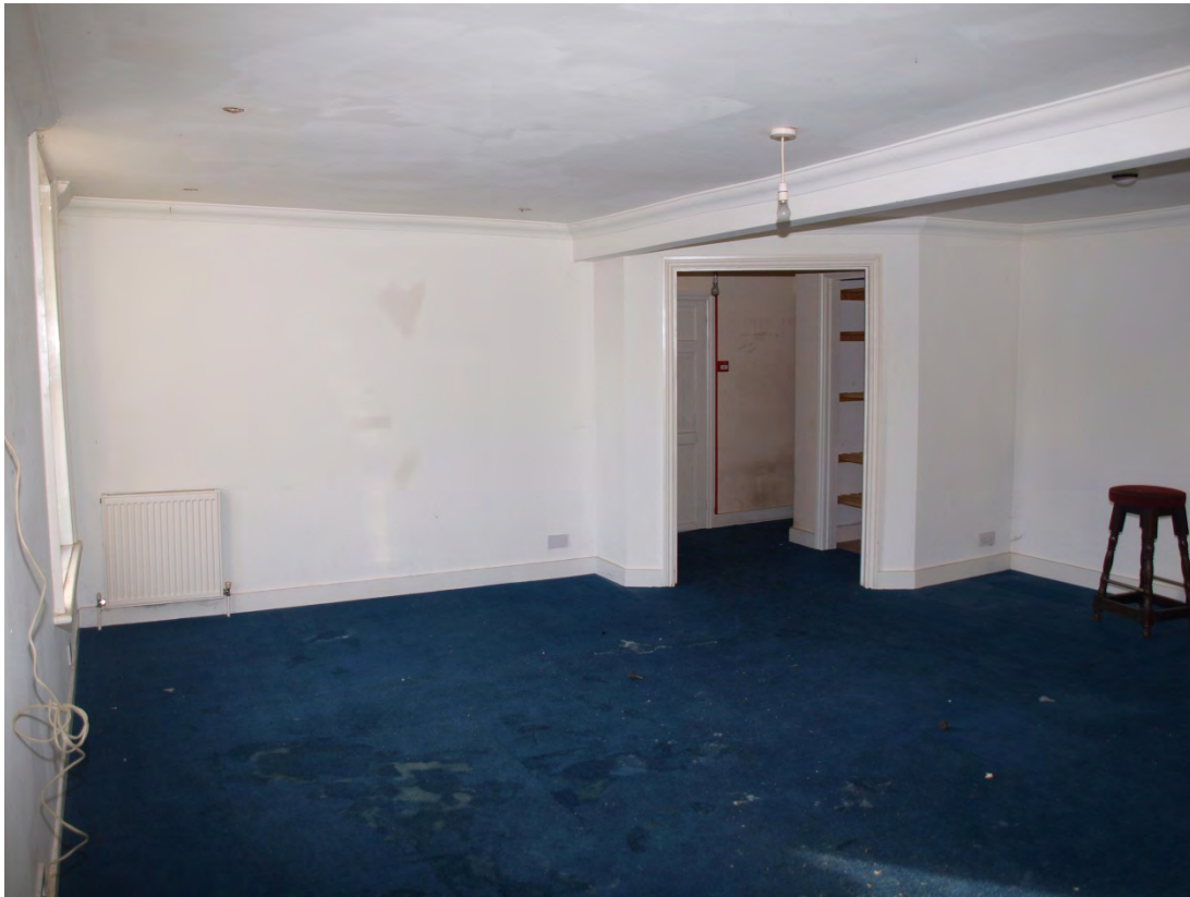
Plate 17: Large room within southern end of principal range, looking south (44)
