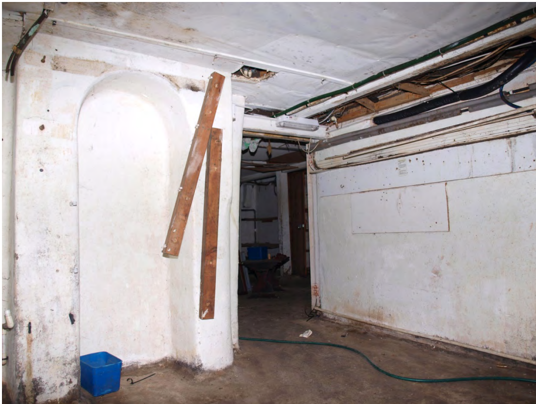
Plate 14: Northern room within cellar, showing base for chimney-stack, looking south-west (36)
