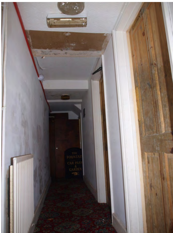
Plate 12: Ground floor corridor showing differences in ceiling level, looking south (28)
