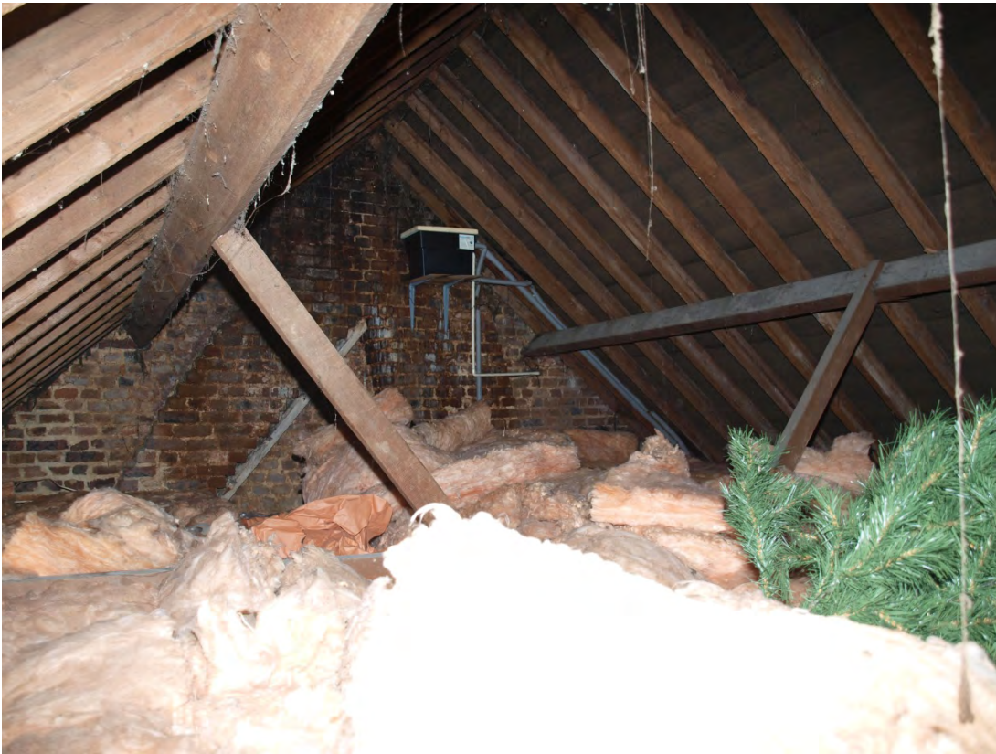
Plate 19: Roof over northern end of principal range, looking north-east (57)
