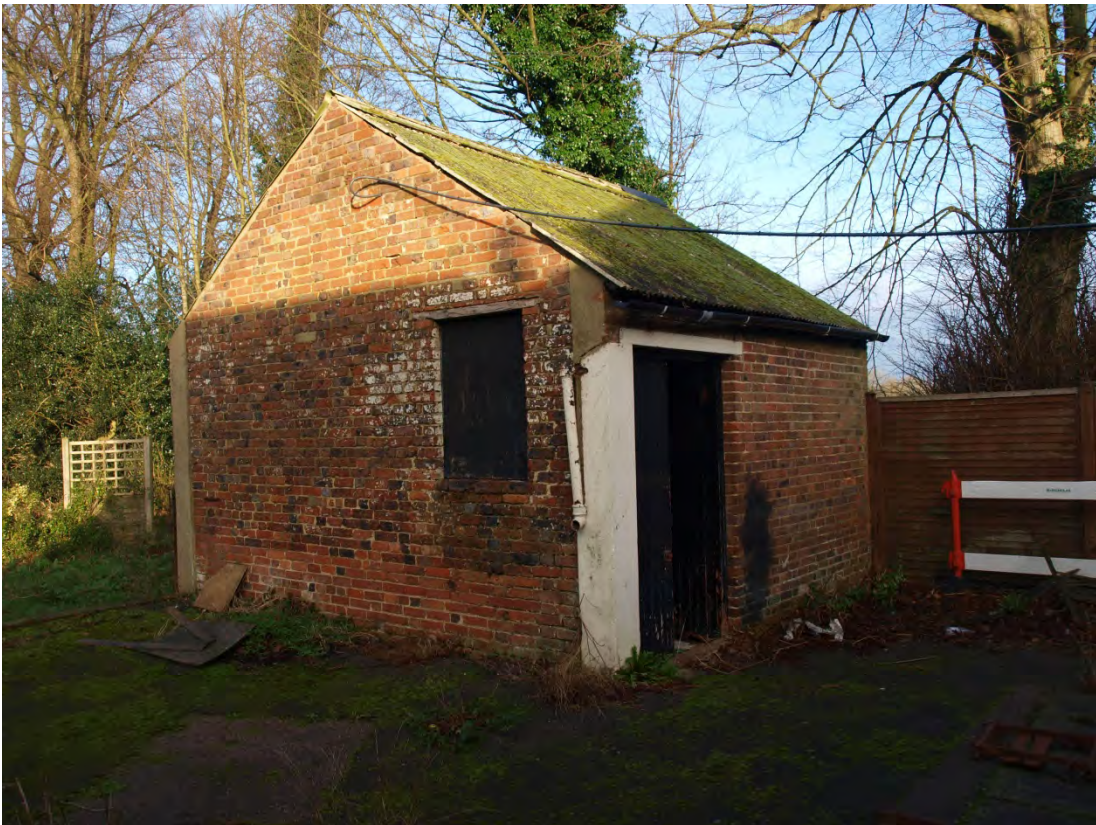
Plate 22: South and east elevations of the outbuilding, looking north-west (13)
