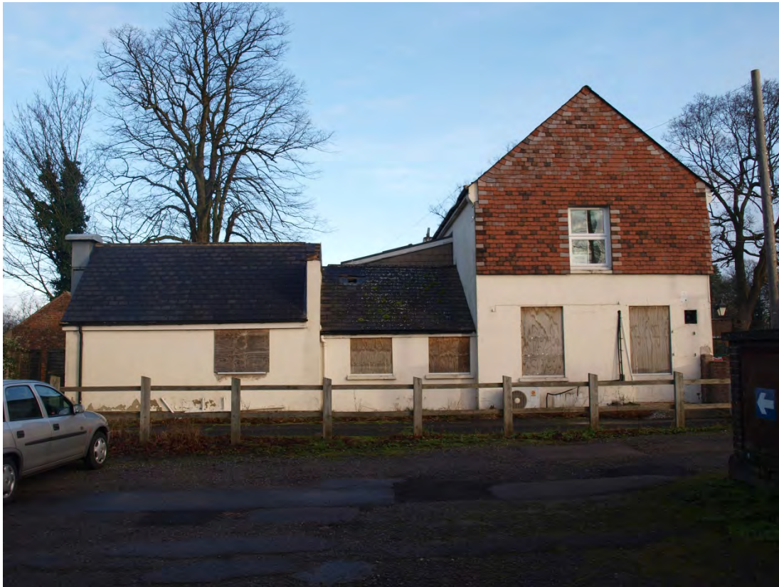
Plate 3: South elevation, looking north (5)
