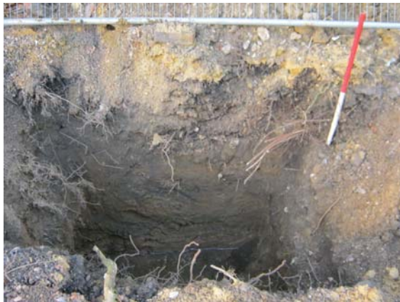
Soakaway 1 facing west
