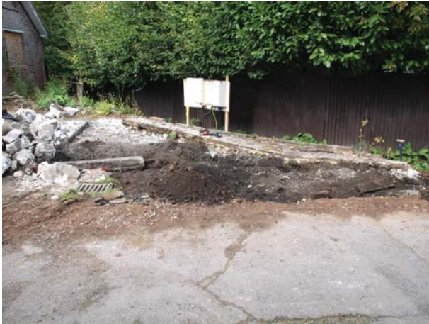
Ground reduction of triangular area with concrete footing [135]
