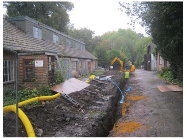
Service trench with Unit 1 in background left (looking north east)
