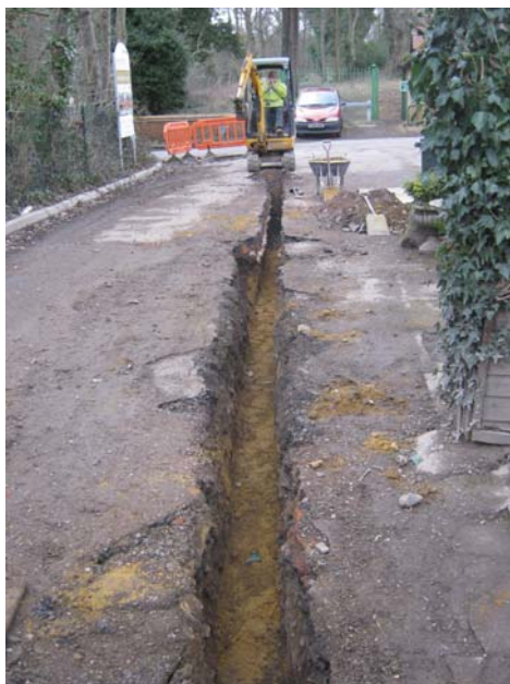
Northern end of service trench (looking north east)
