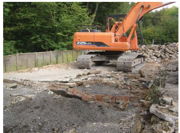
Removal of slab in Unit 1 showing masonry wall [207]
