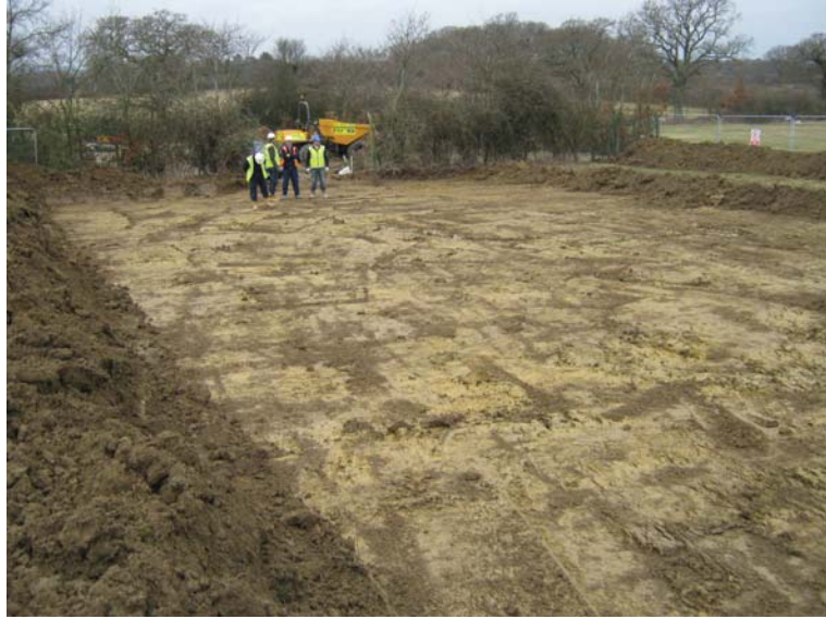
Monitored area looking west
