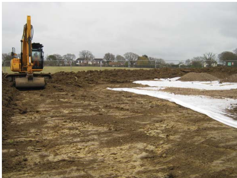
Laying terram over stripped area
