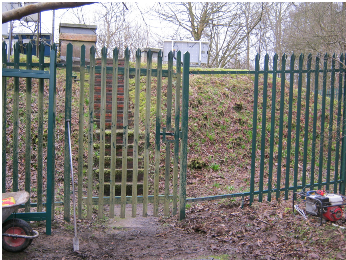
South-east facing view of monitored works
