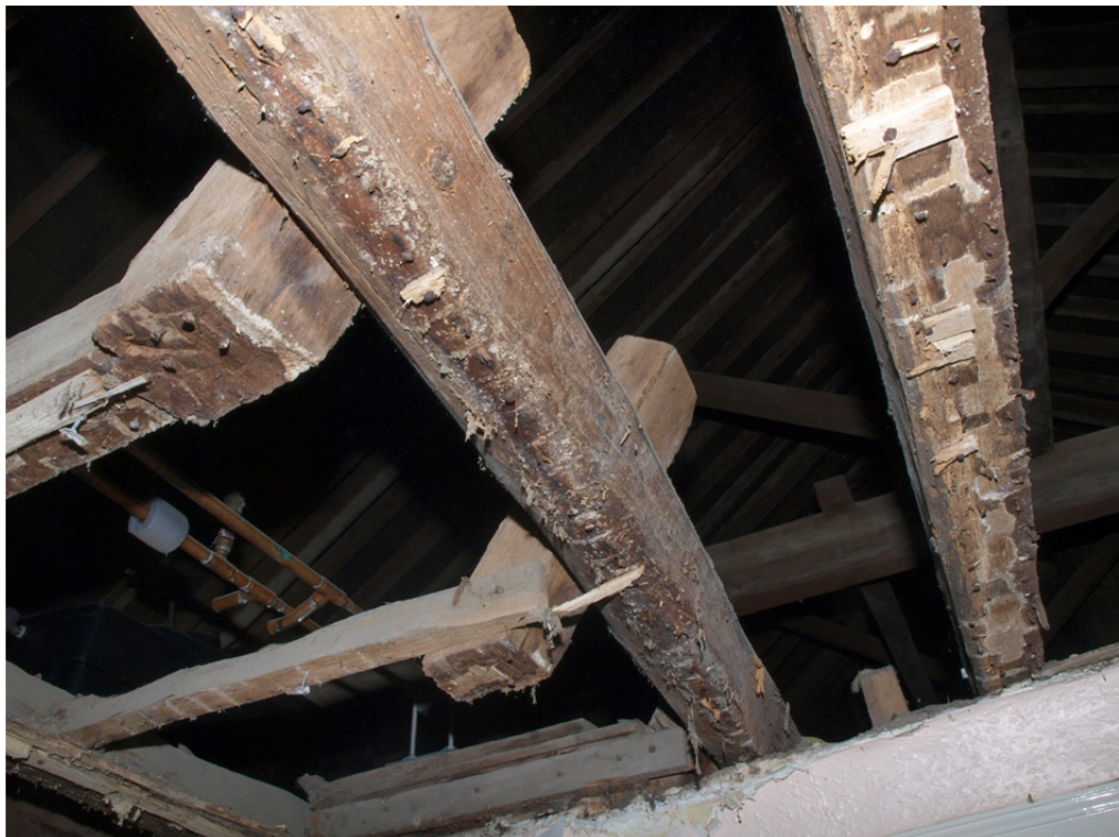
Plate 2: truncated rafters over the first floor staircase shows continuation of the Phase 1 roof
