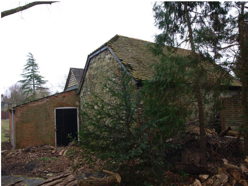
The north elevation
