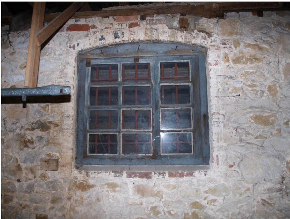
Roof of Block 1 facing south
