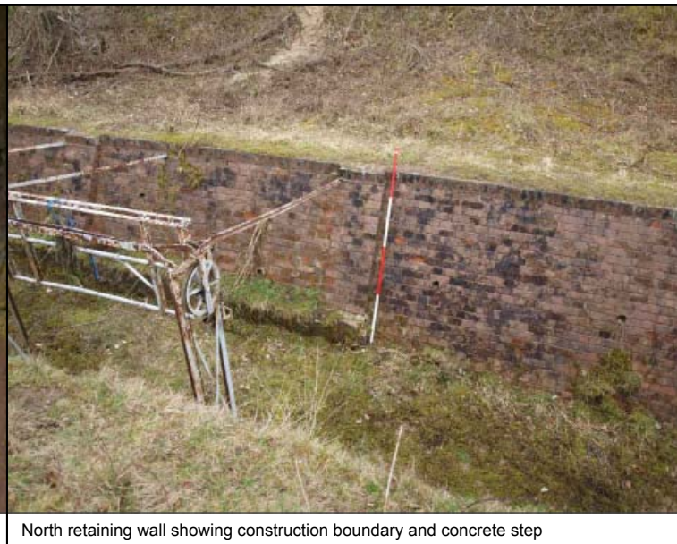
North retaining wall showing construction boundary and concrete step
