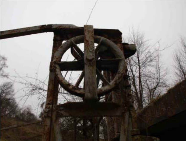
Target frame hoist wheel
