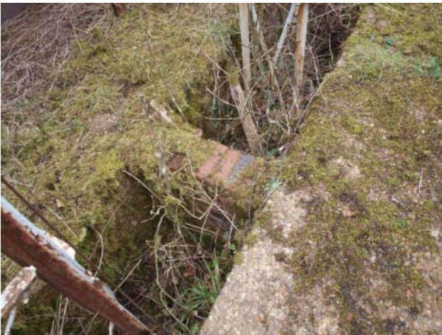
Brick dividing wall within target troughs
