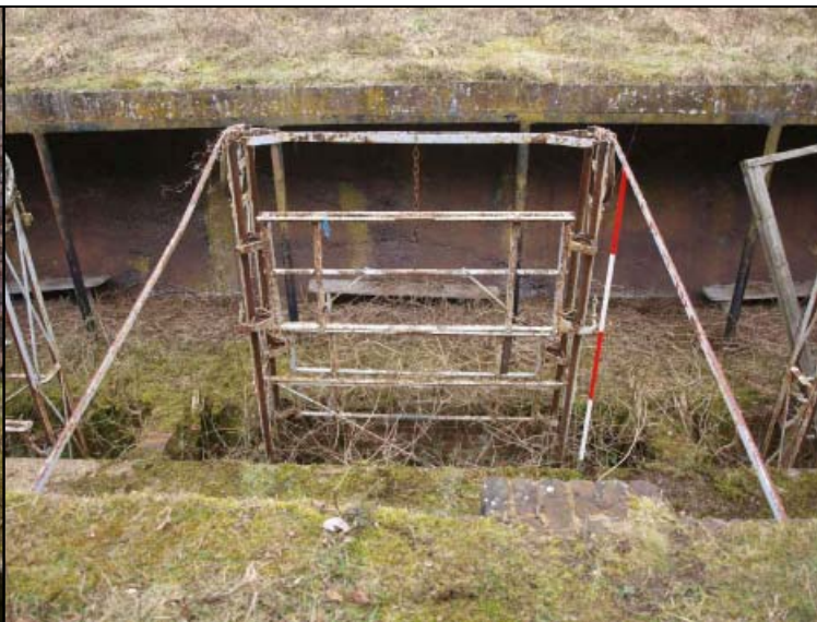
Target frame (Hythe pattern), showing carriages and securing bars, looking north
