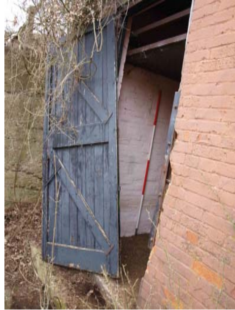
Door to target store and suspended mesh ceilings
