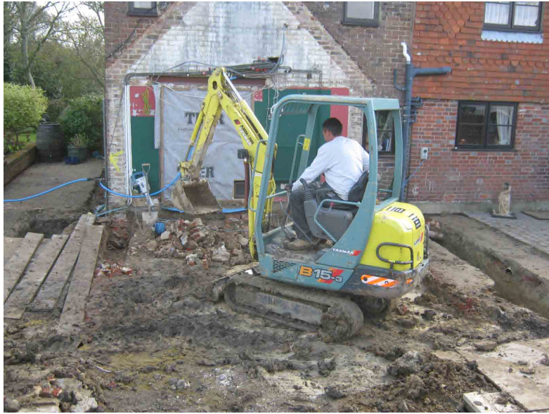
Extension footings being excavated, looking east
