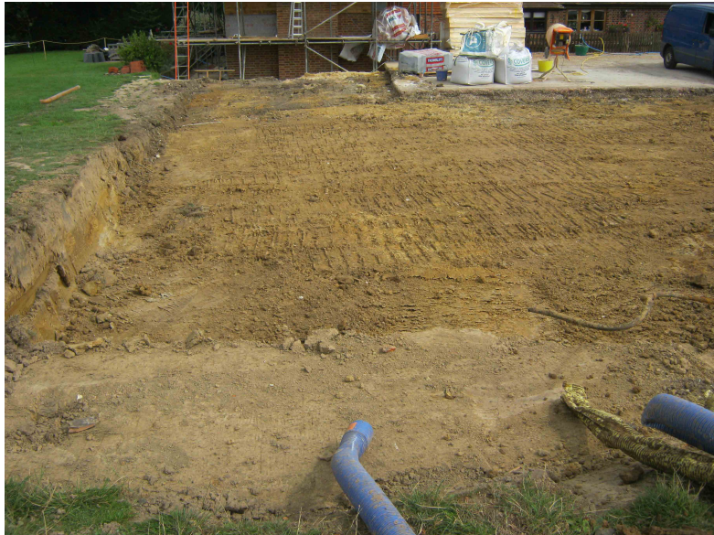
Area of ground reduction, looking east towards completed extension
