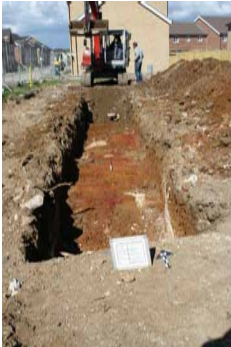
Fig. 4c: Trench 2, facing north
