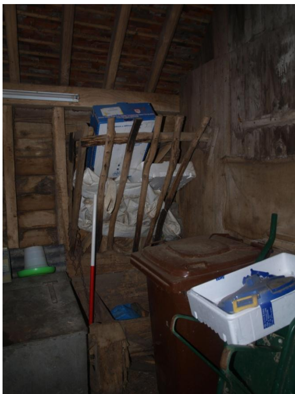
Plate 14: Building 1 – detail of in situ feeding rack and trough
