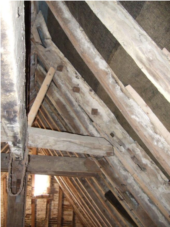
Plate 38: The farmhouse – plate re-used as a rafter shows diamond mortises for window of earlier structure
