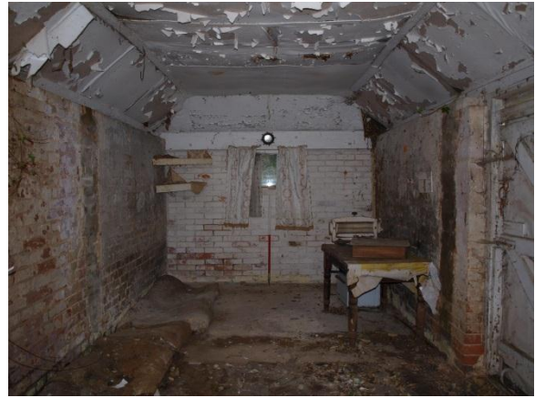
Plate 37: Building 5 – stripped out units
