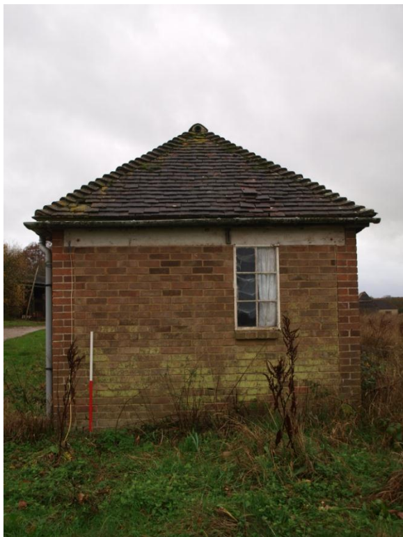
Plate 28: Building 4 – northeast end elevation
