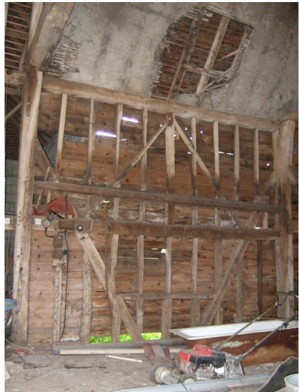
Plate 61: The Barn – rear wall with cleats to support oast floor joists
