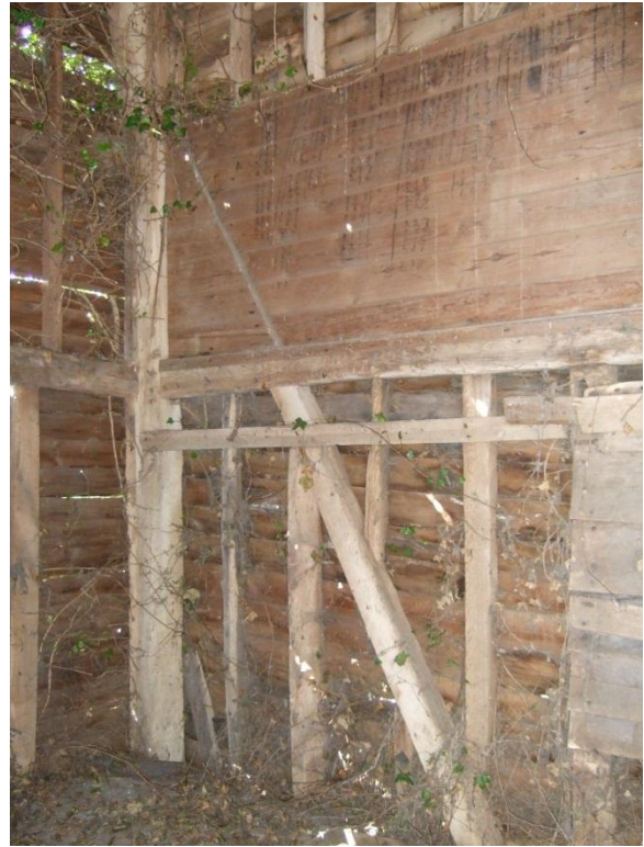
Plate 51: The Barn – Period A wall construction, straight brace halved past external face of side girt
