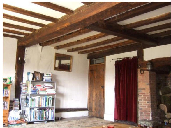
Plate 41: The farmhouse – joists and girder in floor construction over the hall
