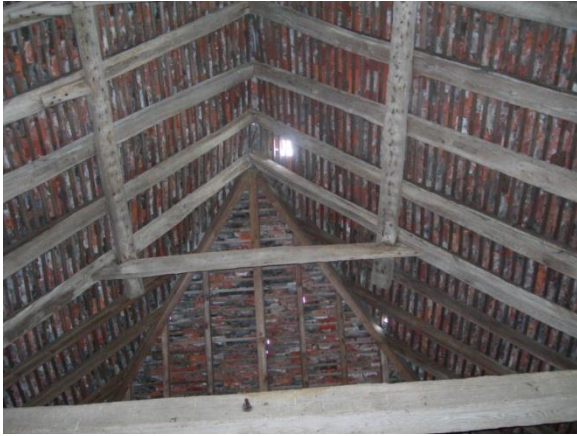
Plate 9: Steddenden Barn – hipped roof terminal construction
