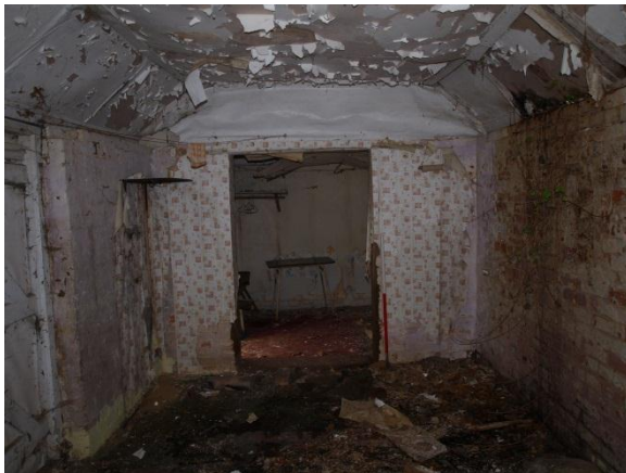
Plate 34: Building 5 – interior finishes
