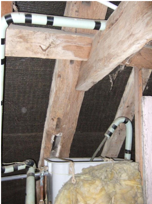
Plate 44: The farmhouse – Period B clasped side purlin roof detail
