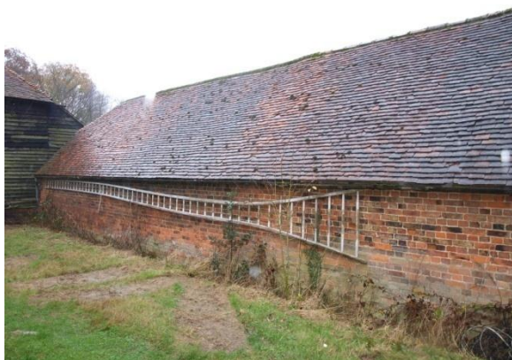
Plate 16: Building 2 – rear northeastern elevation
