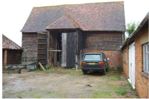
Plate 55: The Barn – external view showing gabled roof terminals
