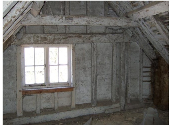
Plate 39: The farmhouse – Period-1 roof truss detail
