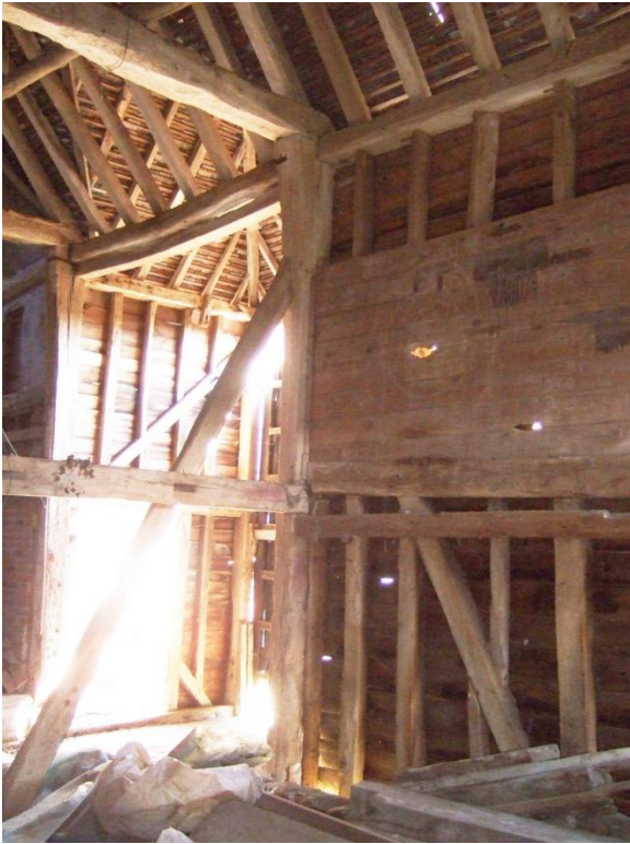
Plate 50: The Barn – Period A normal assembly of tie-beam, wall plate and post
