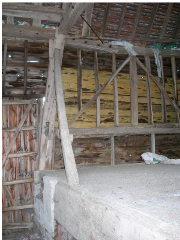
Plate 6: Steddenden Barn – detail of wall construction with straight raking shores
