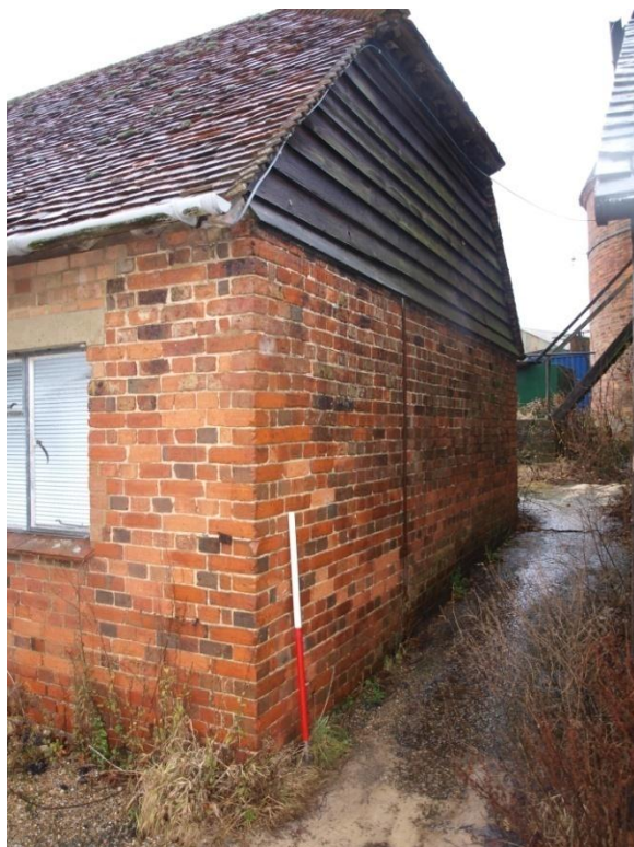
Plate 18: Building 2 – the southeast end elevation
