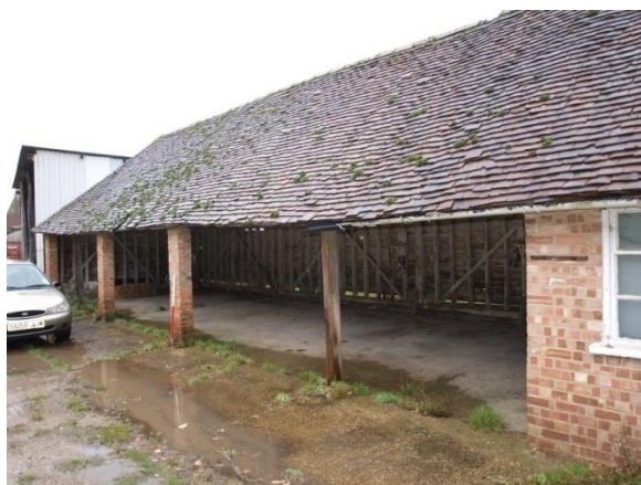
Plate 20: Building 3 – the principal southeast elevation
