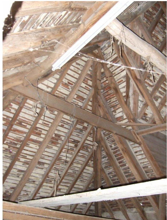
Plate 69: The Oast – Period A northern hip in situ
