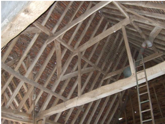
Plate 56: The Barn – roof construction with wind braces
