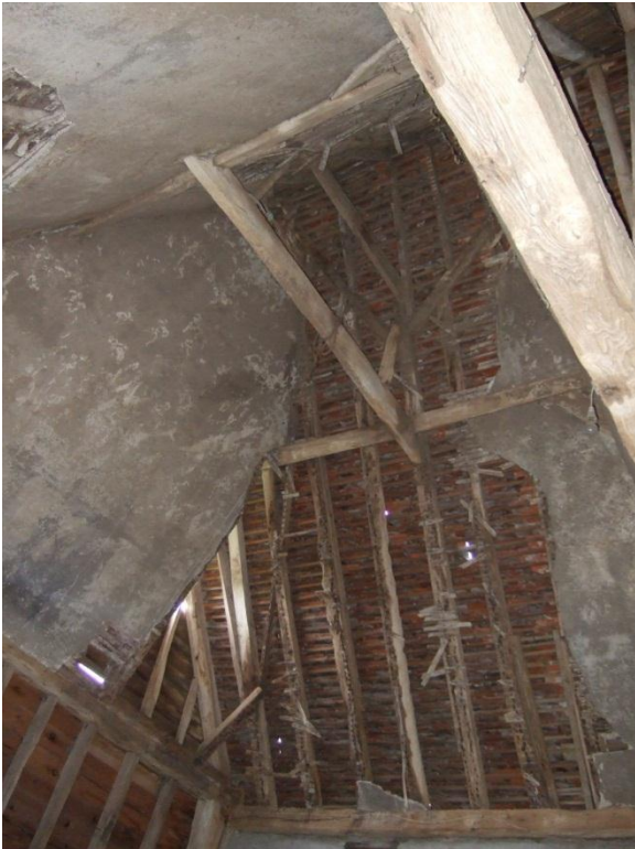
Plate 62: The Barn – supports for flue and cowl
