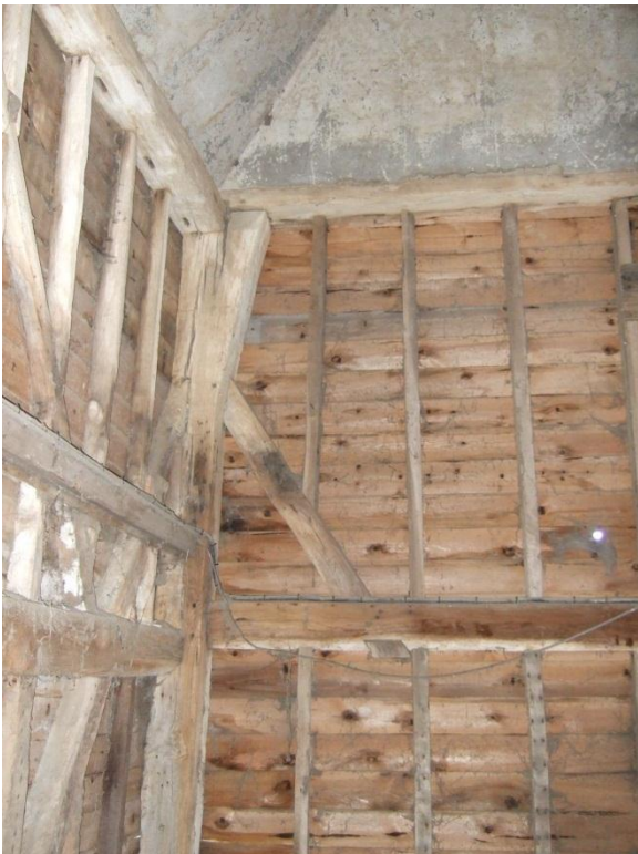
Plate 52: The Barn – Period A wall construction detail with stave holes on plate soffit
