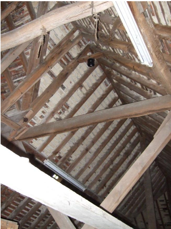
Plate 68: The Oast – Period A southern high-set collar retained but hip removed
