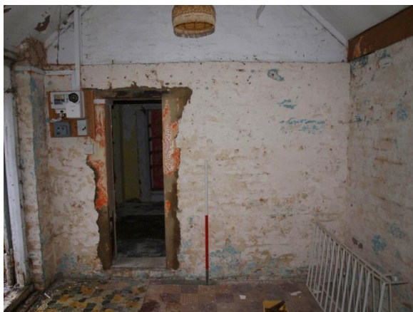
Plate 30: Building 4 – breeze-block partition over brick base
