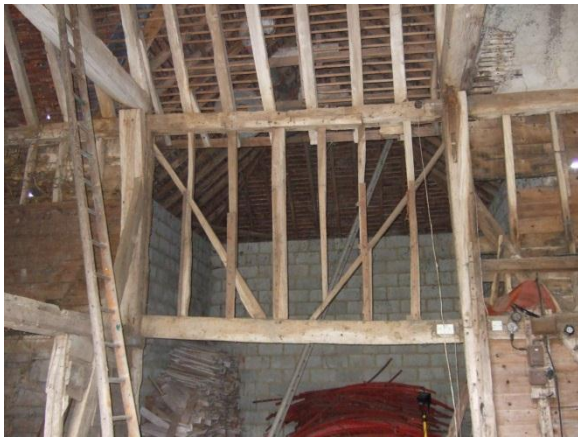
Plate 54: The Barn – half height opening in rear wall
