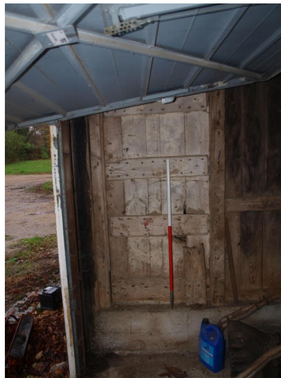
Plate 13: Building 1 – detail of the door into the enclosed southeastern end bay
