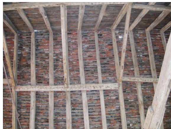
Plate 6: Steddenden Barn – detail of wall construction with straight raking shores
