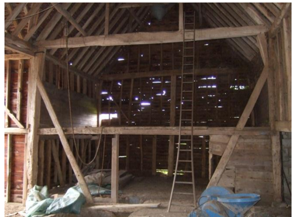
Plate 51: The Barn – Period A wall construction, straight brace halved past external face of side girt
