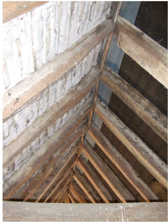
Plate 49: The farmhouse – Period C roof construction
