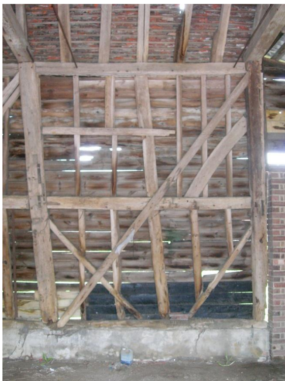
Plate 5: Steddenden Barn – detail of wall construction re-using passing brace
