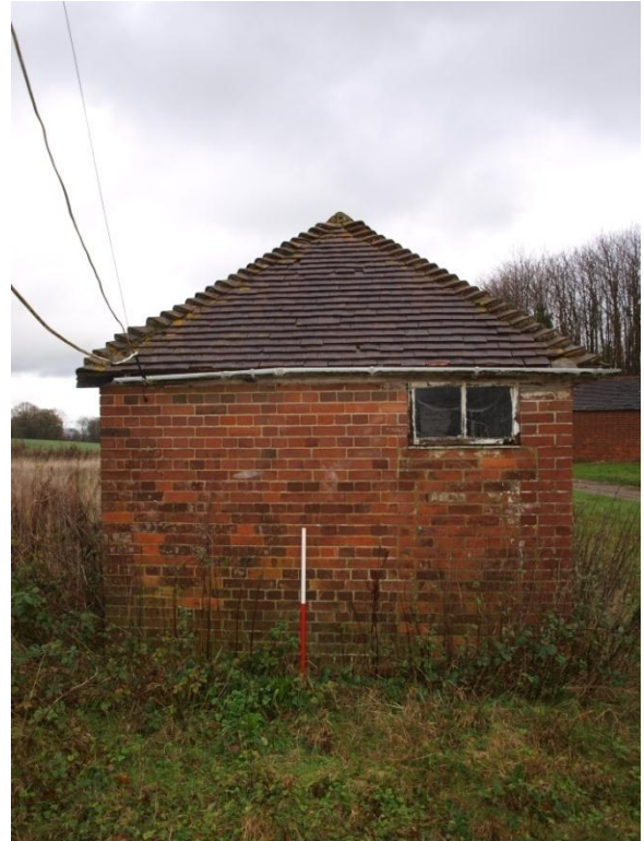
Plate 27: Building 4 – southwest end elevation
