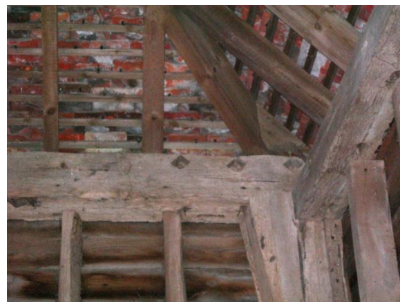
Plate 4: Steddenden Barn – detail of re-used material with diamond mortises for former window opening
