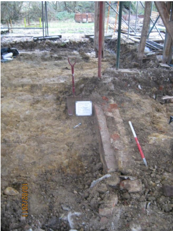
Plate 64: The Barn Watching Brief – the brick footings on the line of truss C-C
