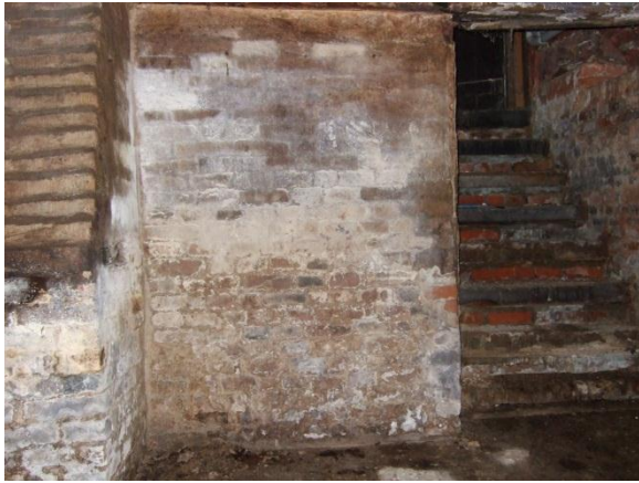
Plate 42: The farmhouse – cellar stairs
