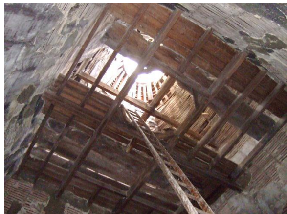
Plate 71: The Oast – roundel brick construction
