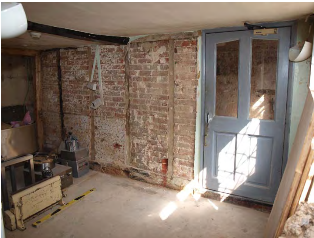
Plate 17: Room 1.04, looking north
