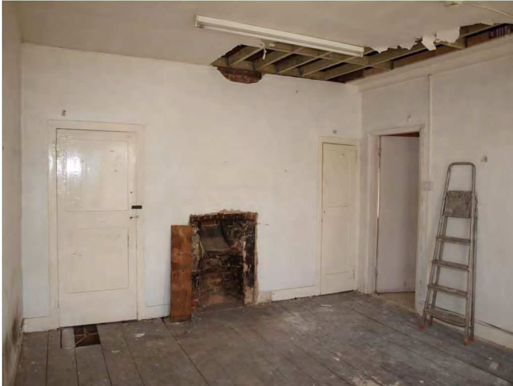
Plate 9: Room 2.02, looking north-east
