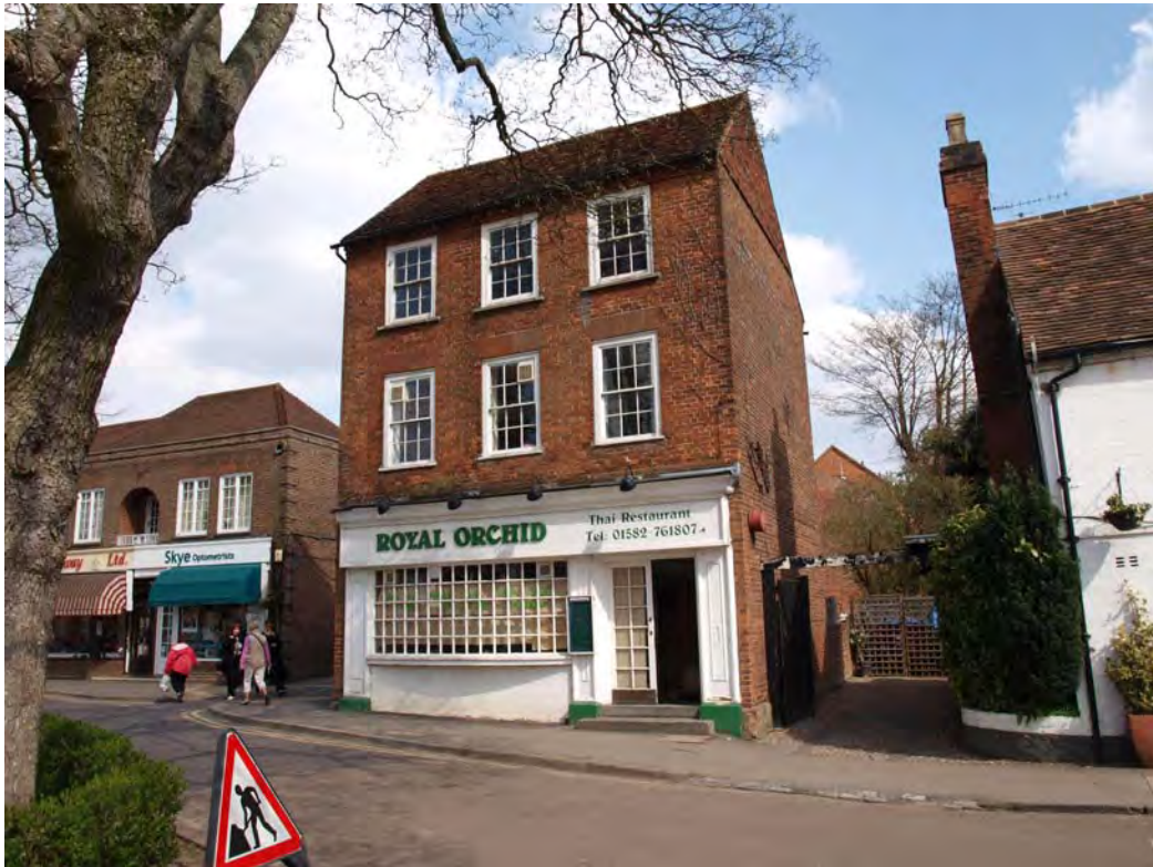
Plate 2: South-west elevation with modern shop-front, looking north-east
