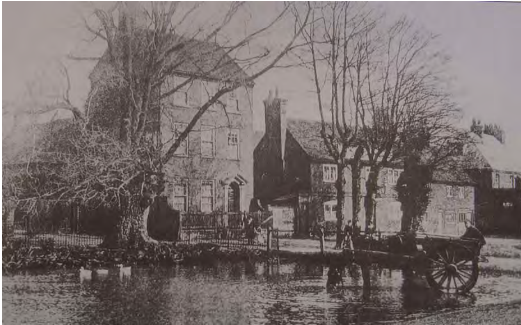
Plate 1: Late-19 th century photograph showing original ground floor arrangement (Source: Brandreth 1996)
