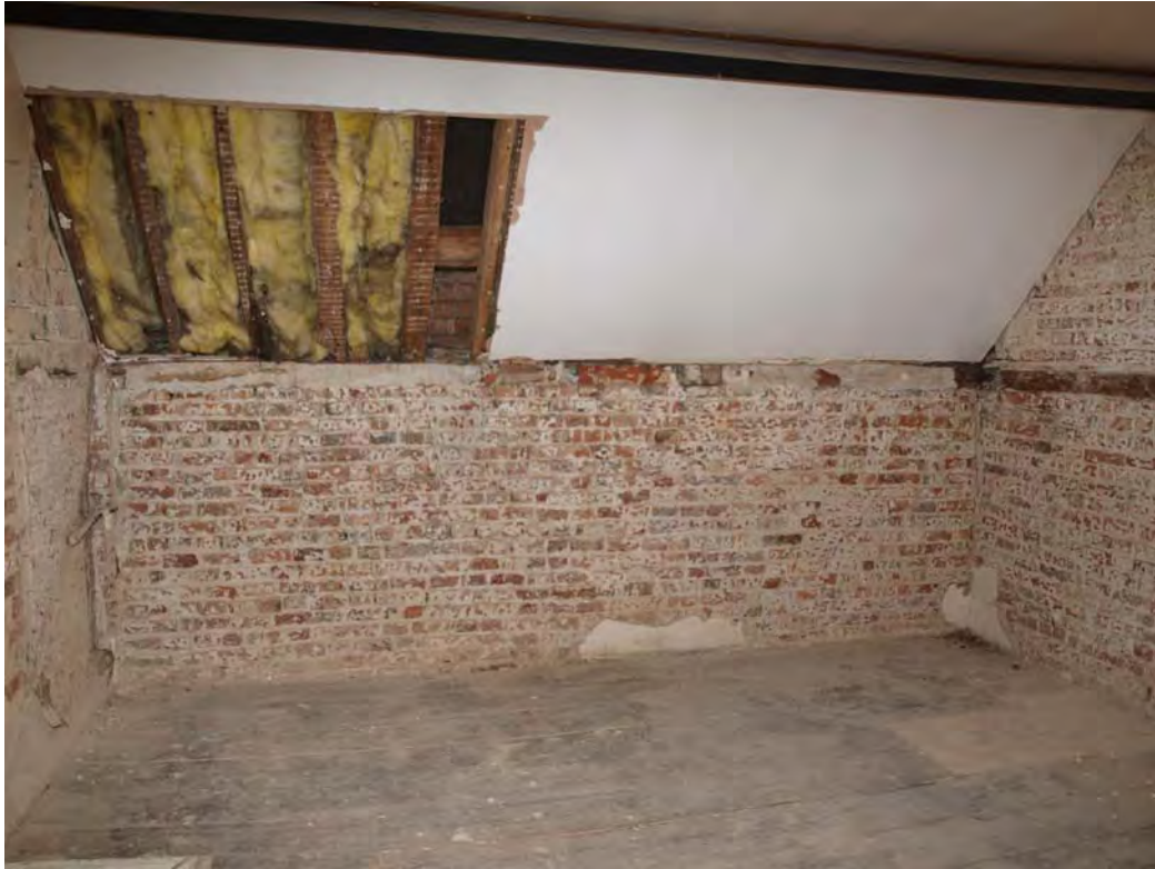
Plate 21: North-west wall of Room 1.05, looking north-west
