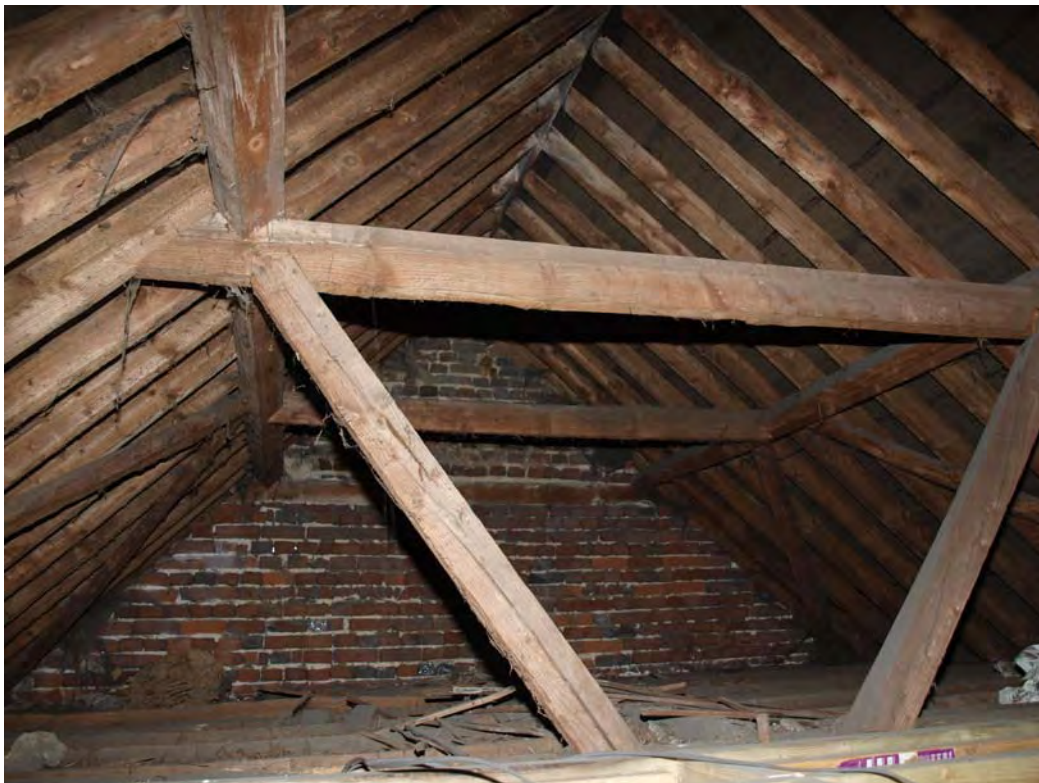
Plate 10: Roof above Unit 1, looking south-east
