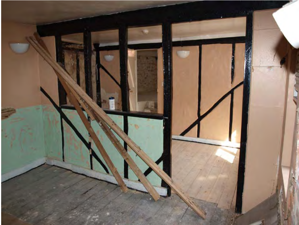
Plate 19: Rooms 1.03 and 1.04, looking north
