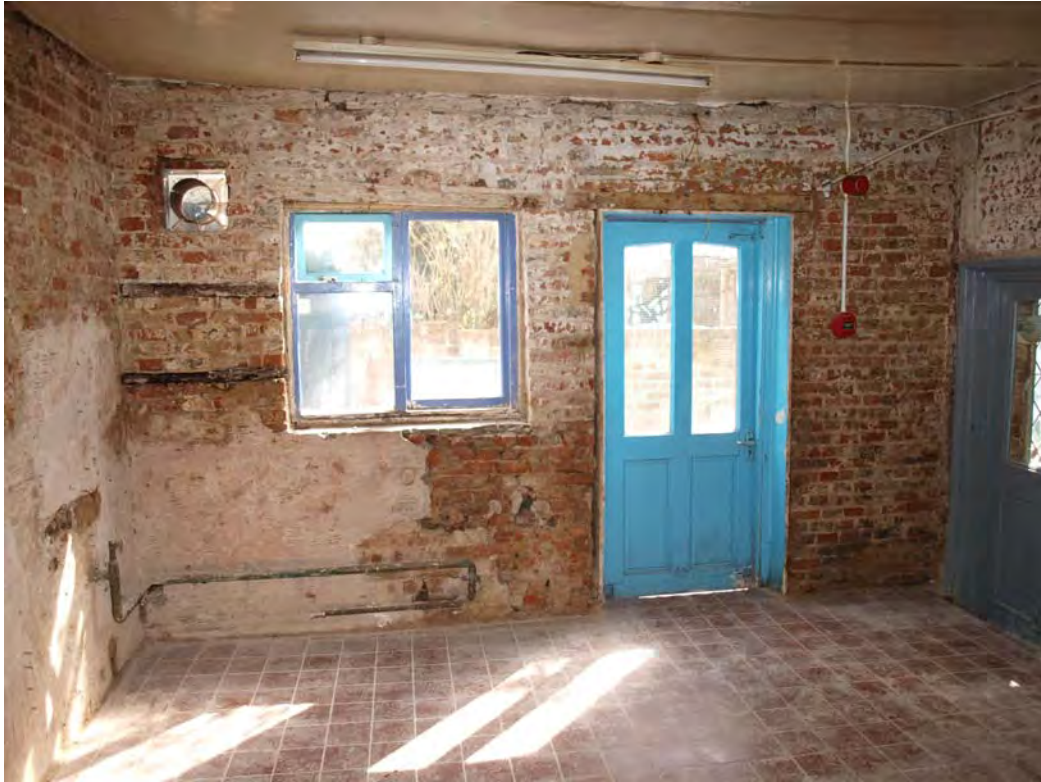
Plate 23: South-east wall of Room G.05, looking south-east
