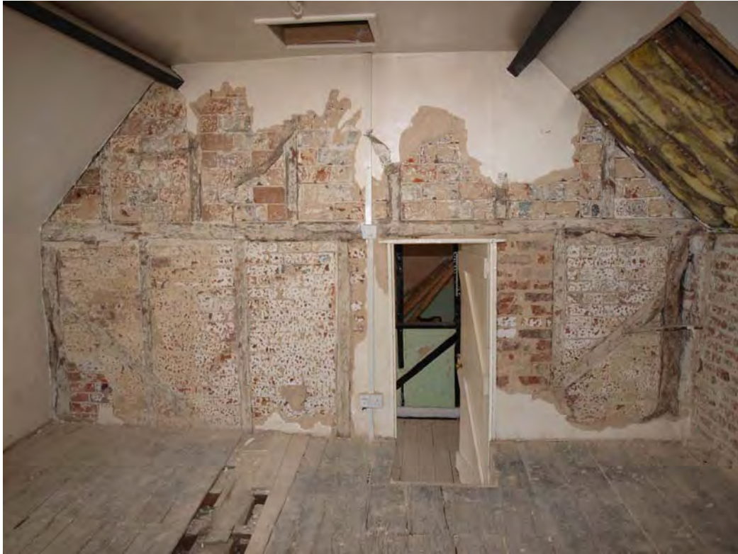
Plate 13: Unit 2 wall-framing, viewed from Room 1.05, looking south-west
