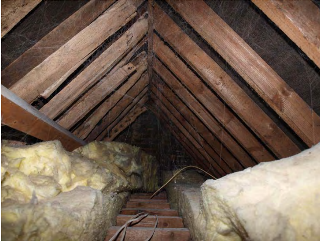
Plate 25: Early rafters within roof over Unit 3, looking north-east
