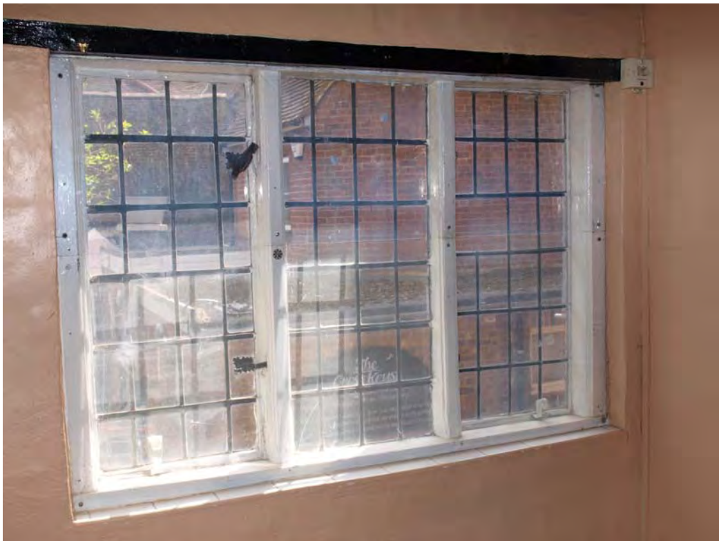
Plate 20: Window on south-east wall of Room 1.04
