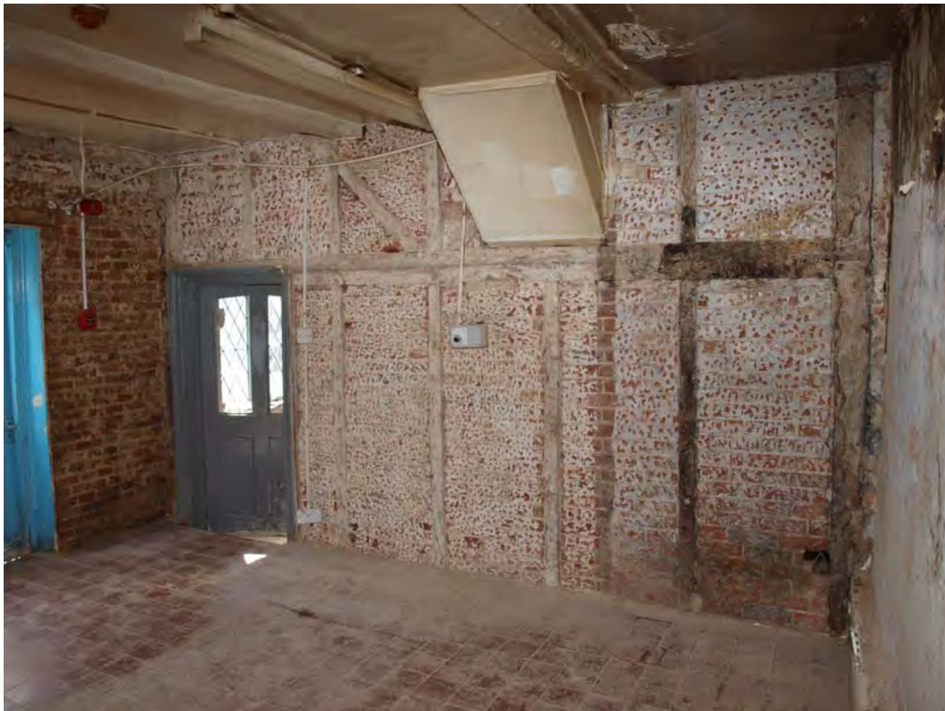
Plate 12: Unit 2 wall-framing, viewed from Room G.05, looking south-west
