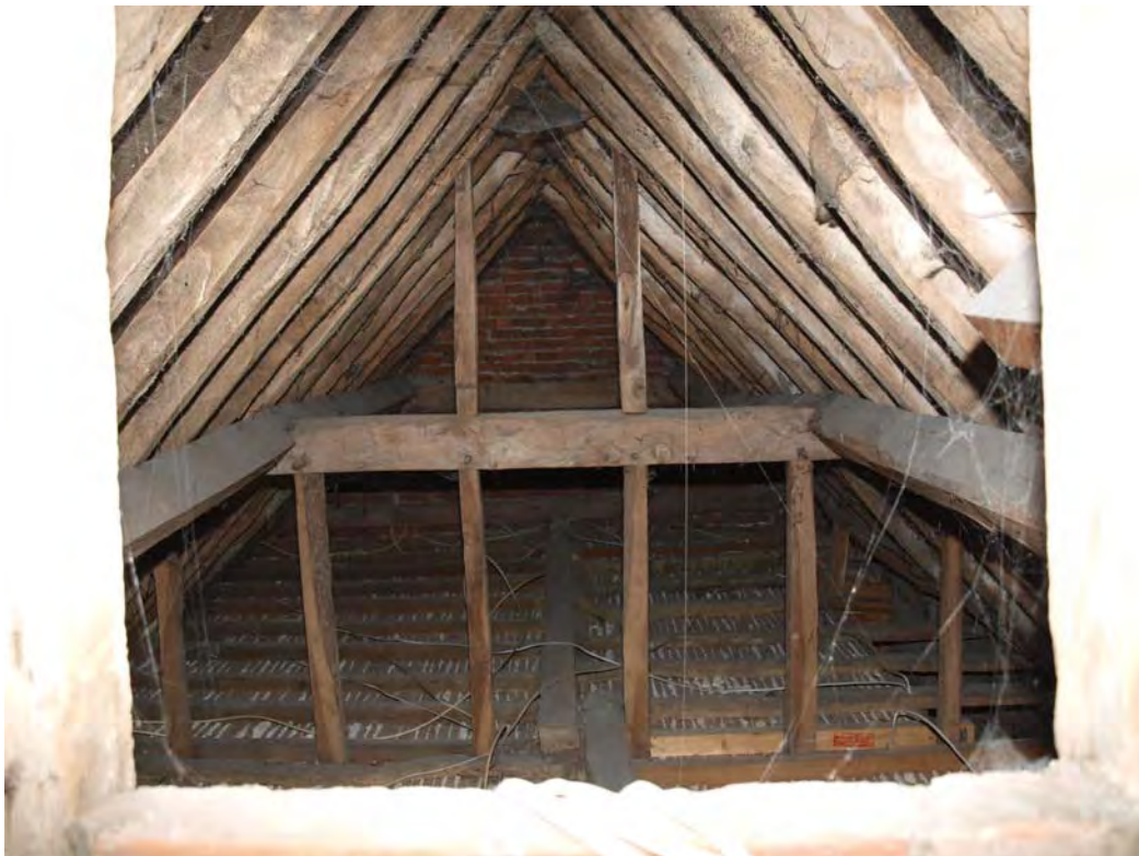
Plate 14: Roof over Unit 2, looking south-west
