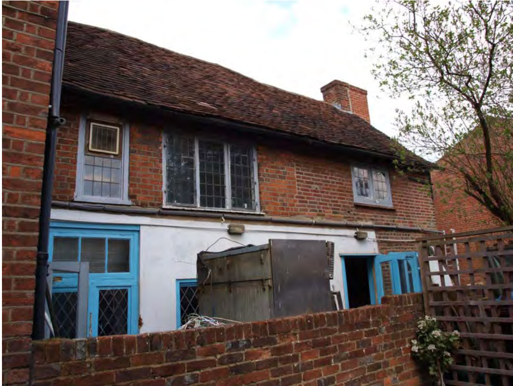
Plate 3: South-east elevation of rear range, looking north
