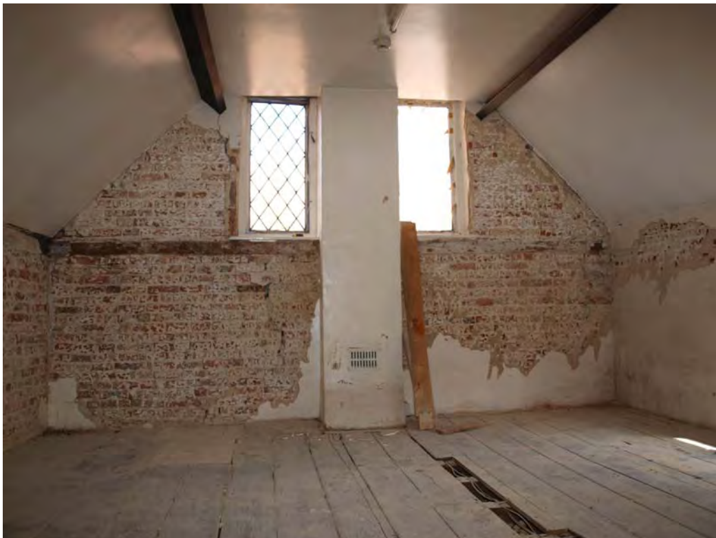
Plate 24: North-east wall of Room 1.05, looking north-east
