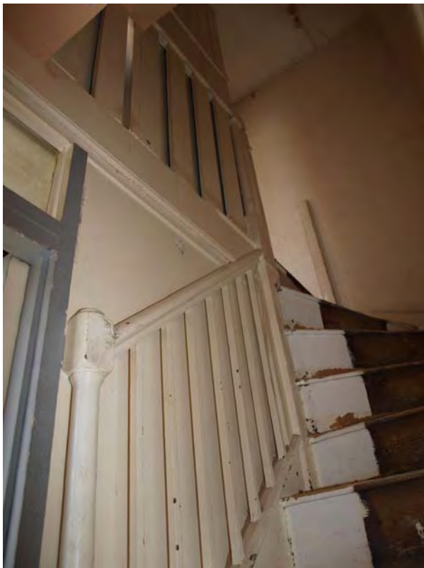
Plate 8: First floor to attic stair, looking north
