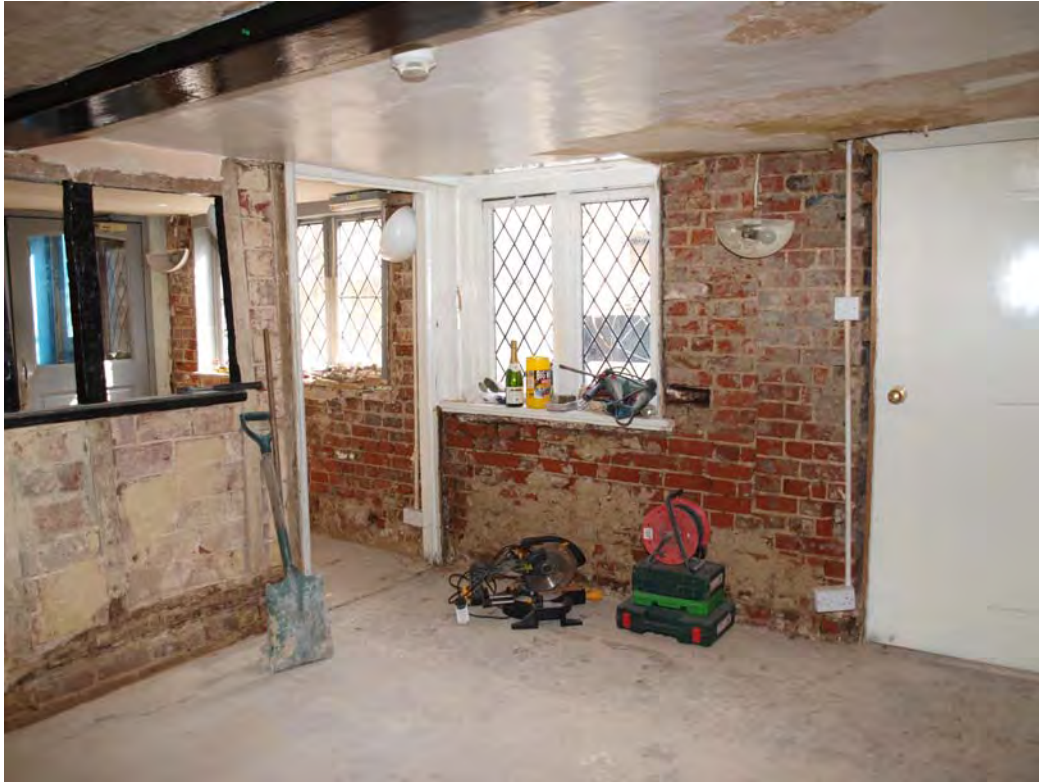
Plate 11: Ground floor south-east wall of Unit 2, showing truncated brickwork at the junction with Unit 3, looking east
