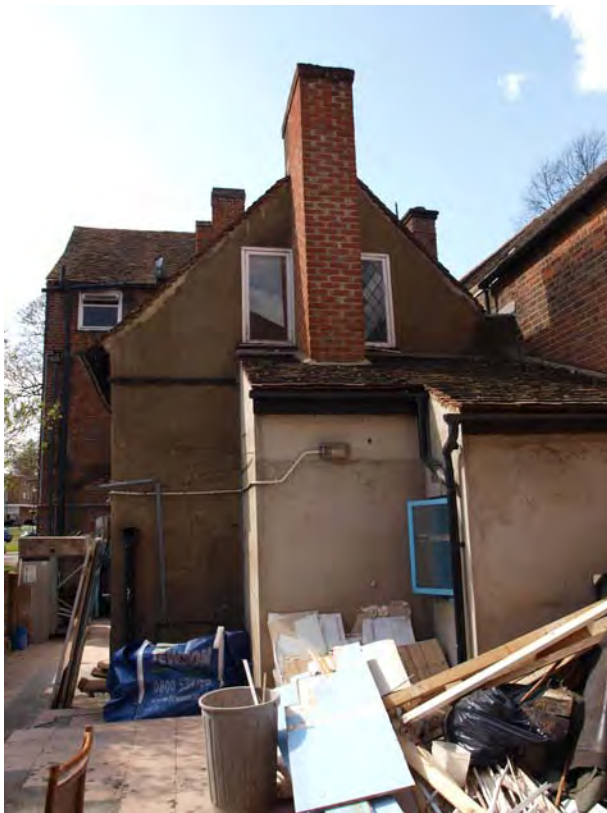
Plate 4: Lean-to (Unit 4) adjoining the north-east gable-end of Unit 3, looking south-west
