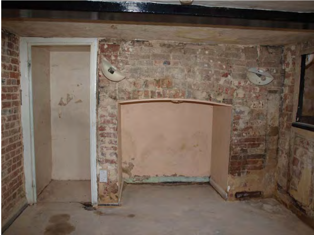
Plate 15: Fireproof safe on north-west wall of Room 1.03, looking north-west
