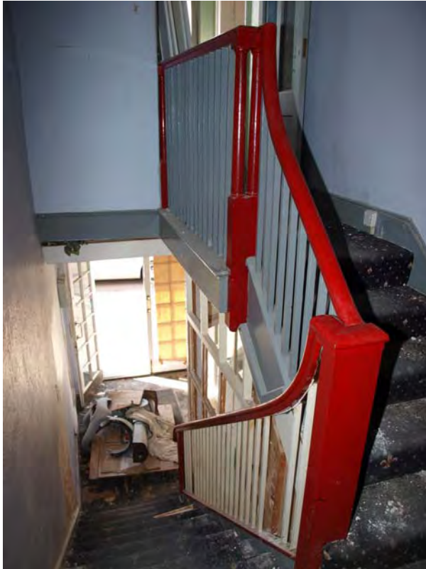
Plate 5: Staircase, looking south-west
