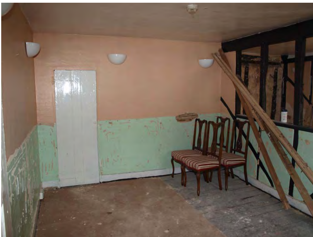
Plate 18: Room 1.03, looking north-west
