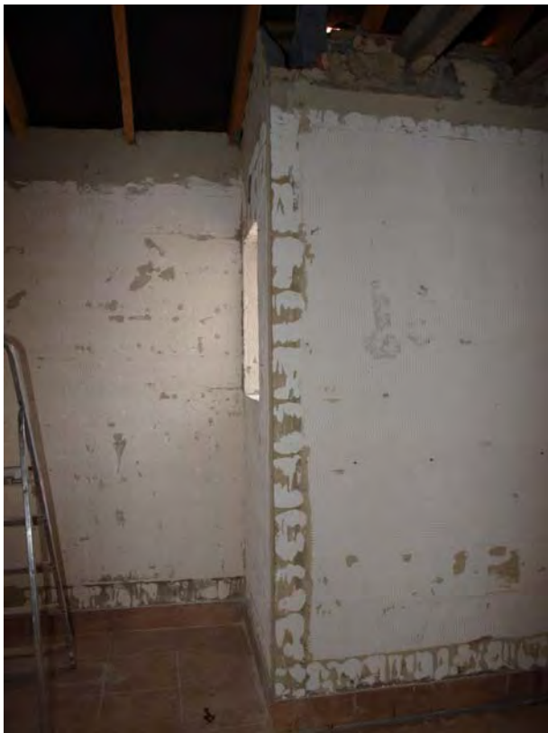
Plate 26: Room G.06, looking north-east
