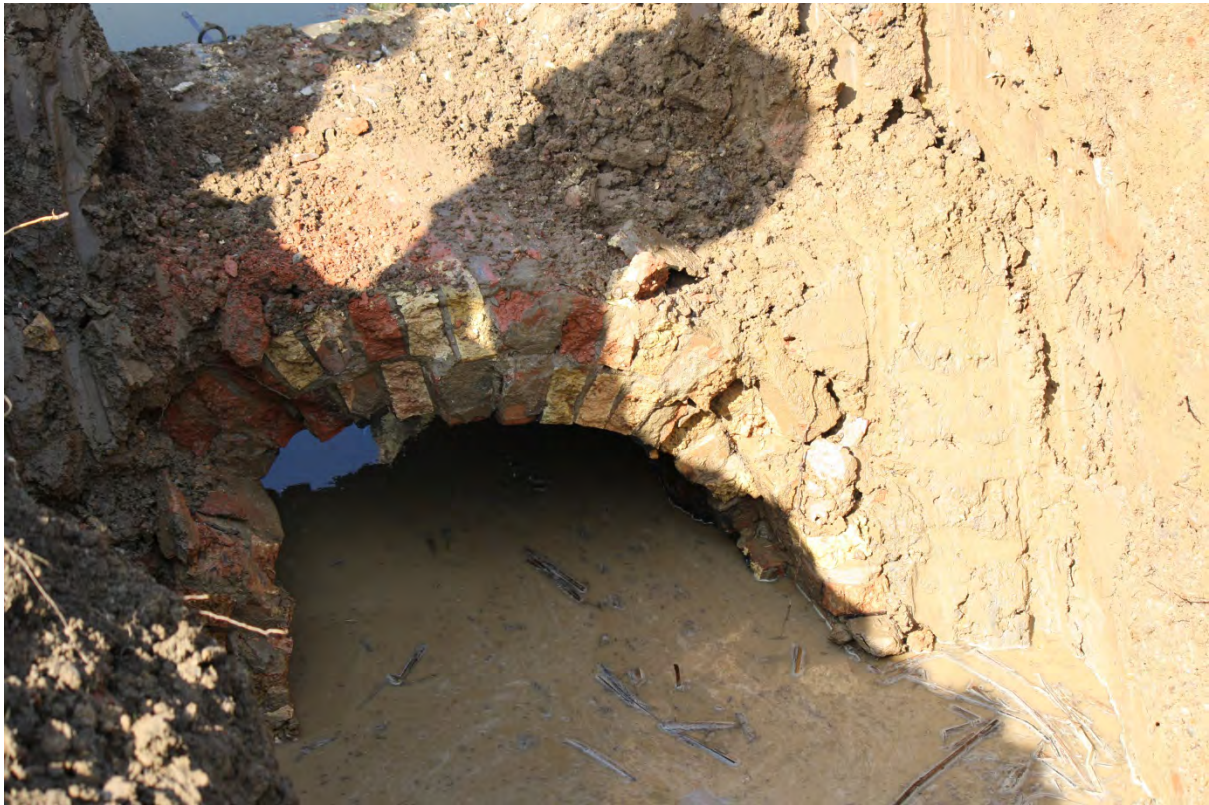
Plate 5: Mixed brickwork at north end of culvert (Stage 6), looking north
