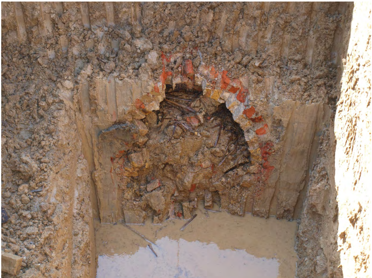
Plate 4: Detail of culvert as seen in north-facing section of Stage 2
