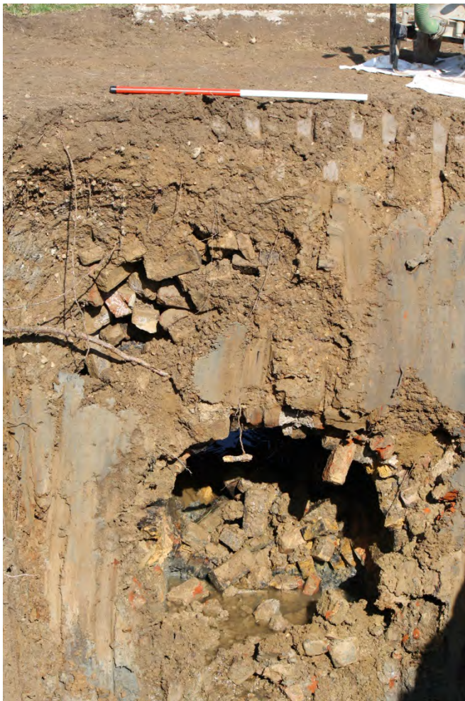
Plate 6: Area of collapse and rubble-filled void (006) visible at Stage 5 of the excavations, looking north
