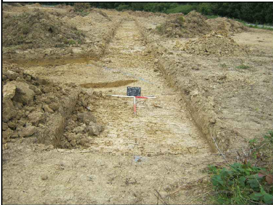
Fig. 12a Trench 18 looking West
