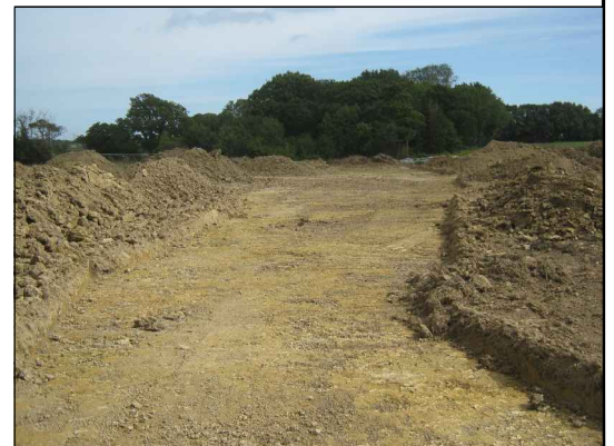
Fig. 16a Mitigation Area A looking West
