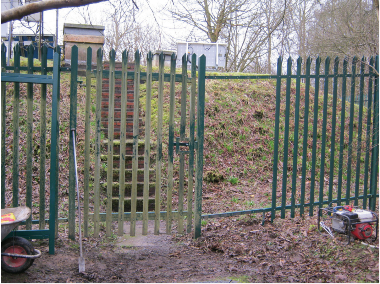
South-east facing view of monitored works
