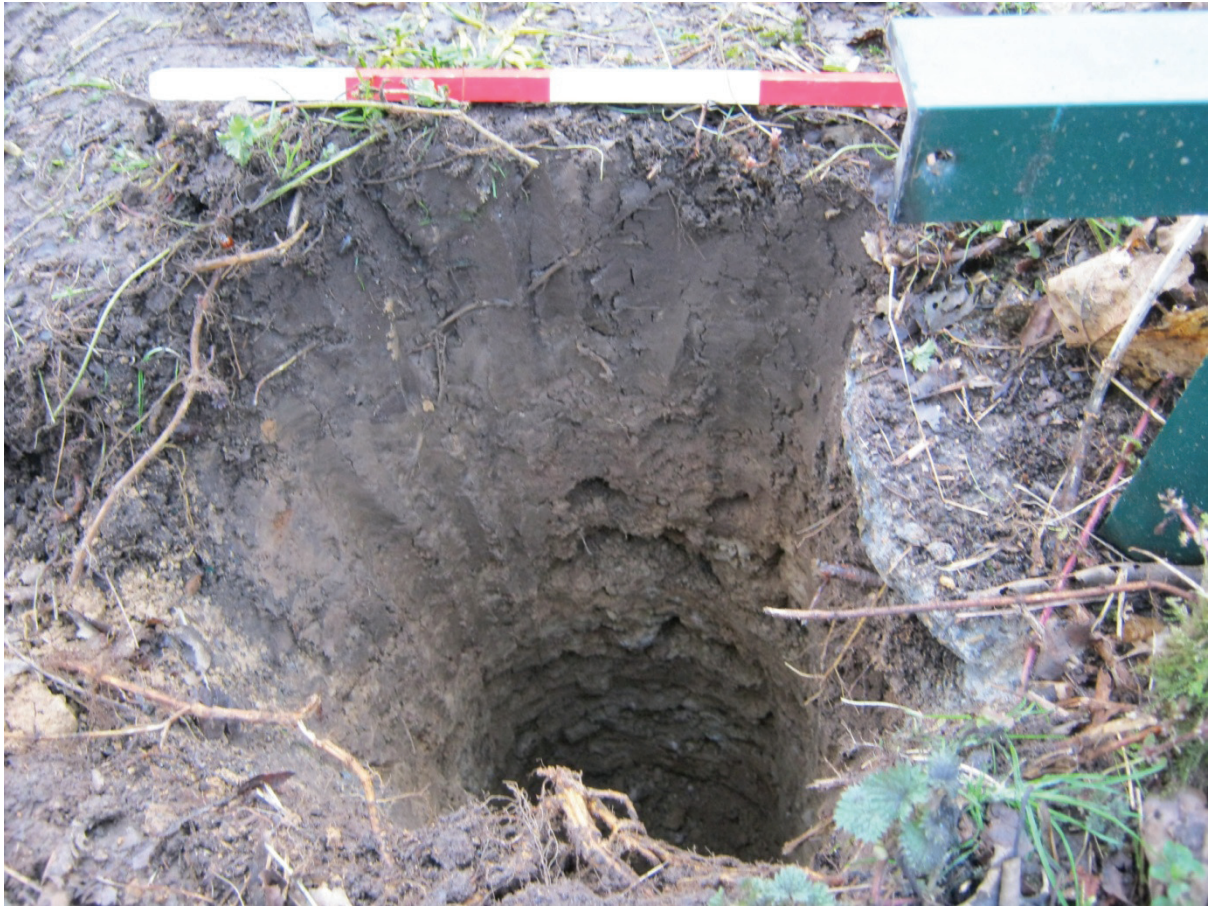
Photograph showing hand excavated posthole for new fence post
