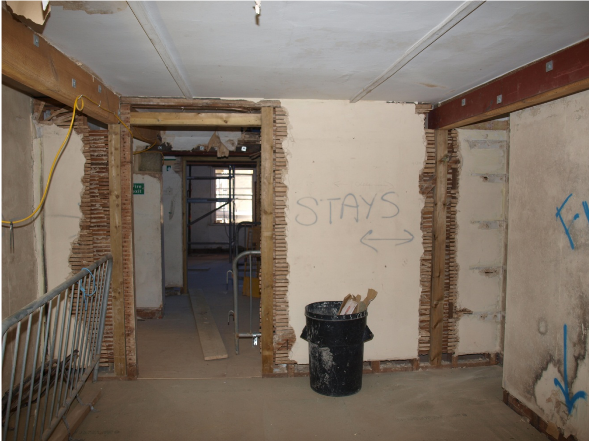
Plate 2: Internal studwork partition wall in Period D western range, looking south
