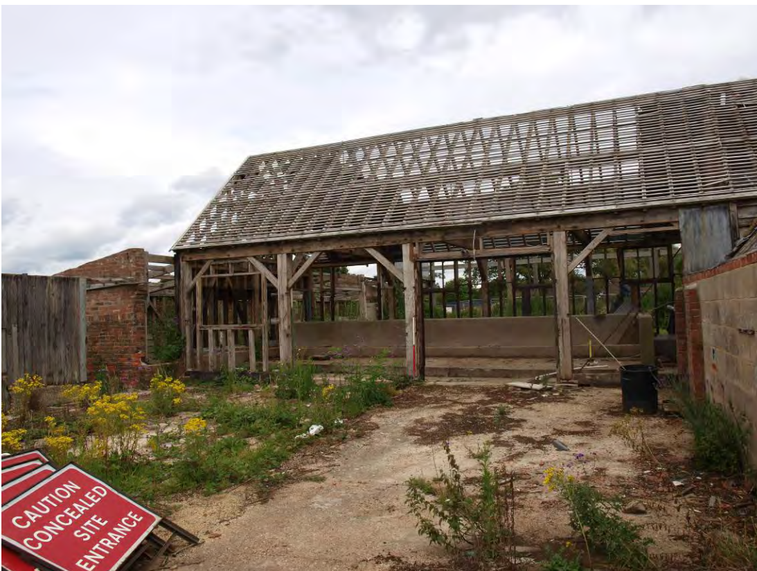
Plate 10: South elevation of Building 2, looking north
