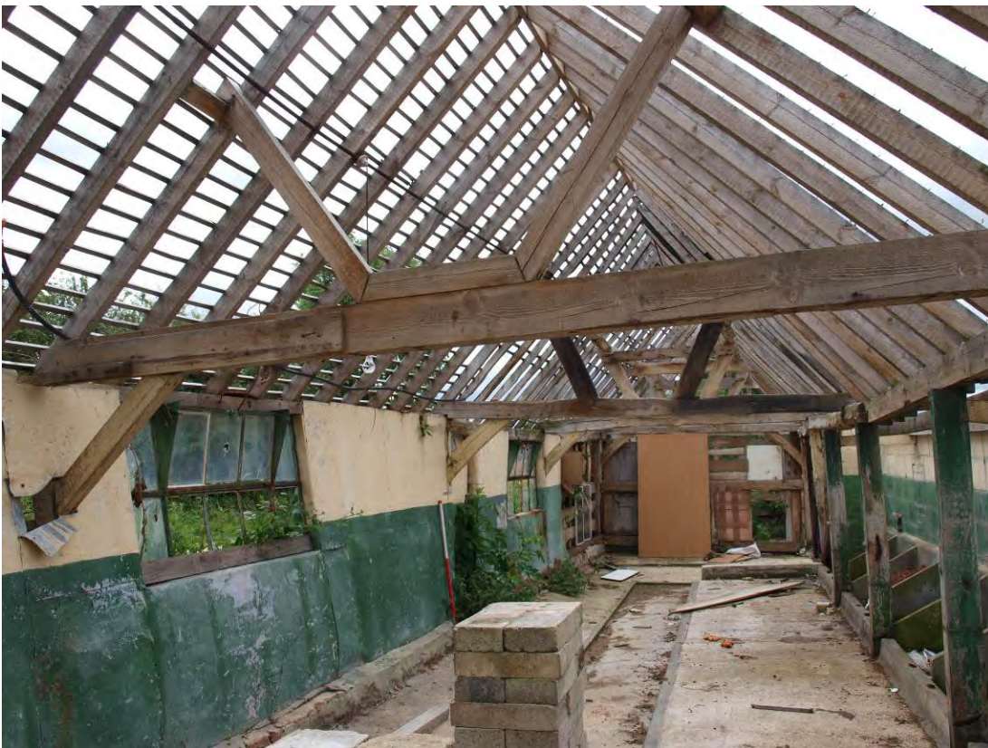
Plate 8: c. 1900 truss to northern section of Building 1, looking south
