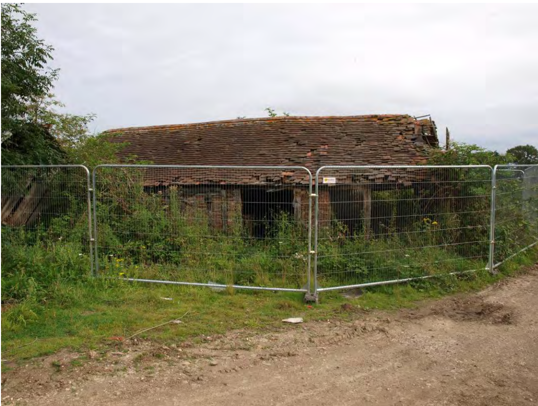
Plate 12: The larger of the two buildings at Hares Hill Farm, looking north
