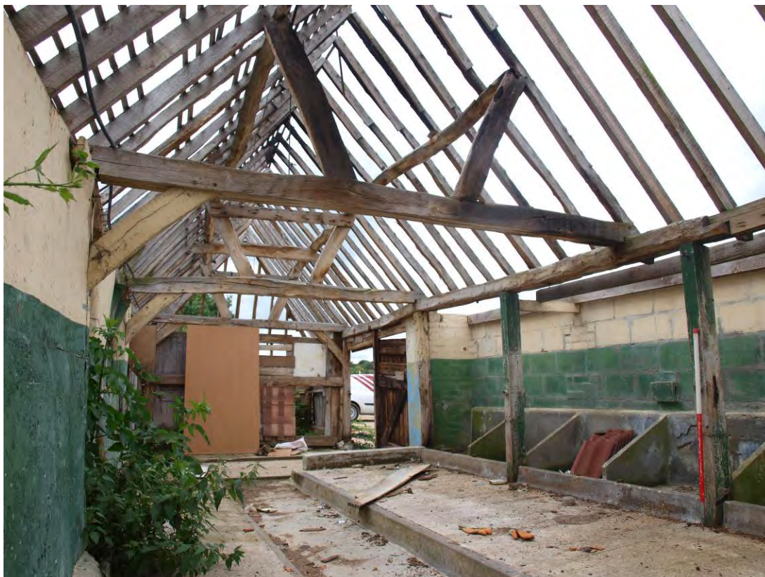
Plate 3: Three surviving bays of original c. 1700 structure (Building 1), looking south
