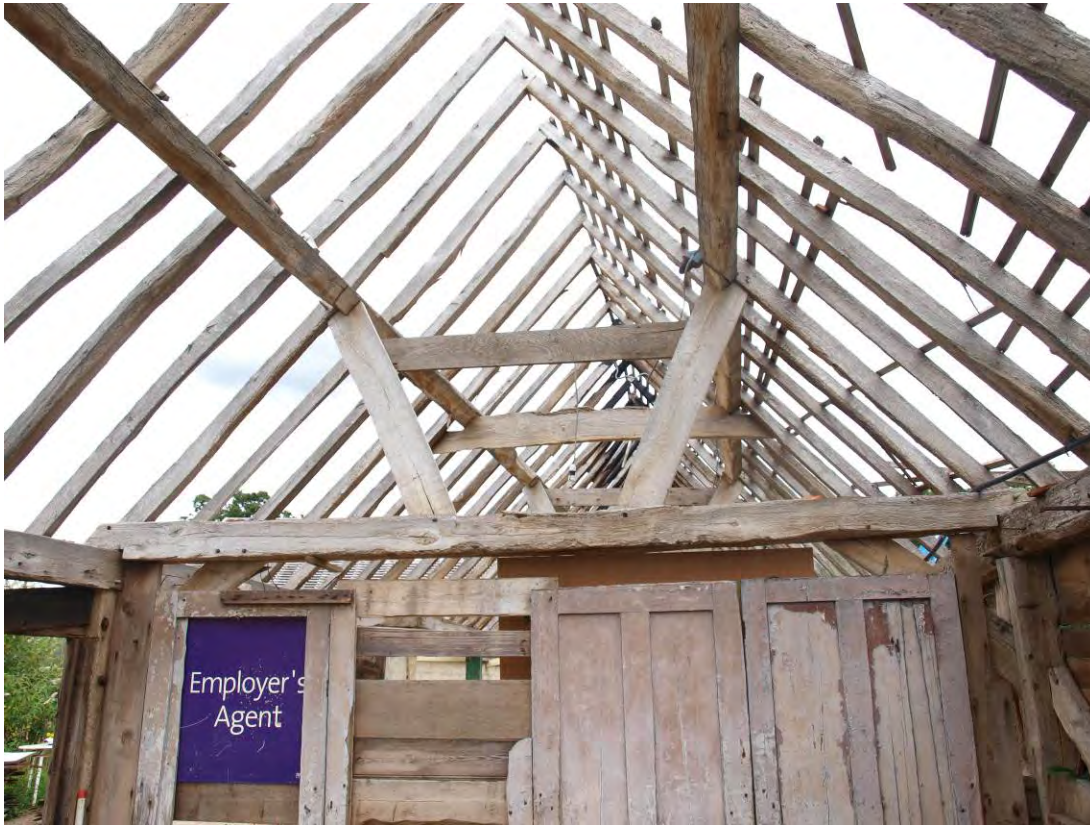
Plate 5: Truss between Bays 1 and 2 (Building 1), looking north
