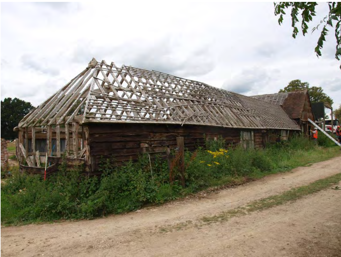
Plate 2: South and east elevations of Building 1, looking north-west
