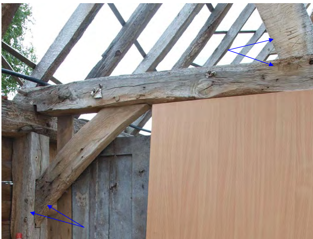
Plate 4: Chiselled carpentry assembly marks (highlighted), upon c. 1700 frame of Building 1
