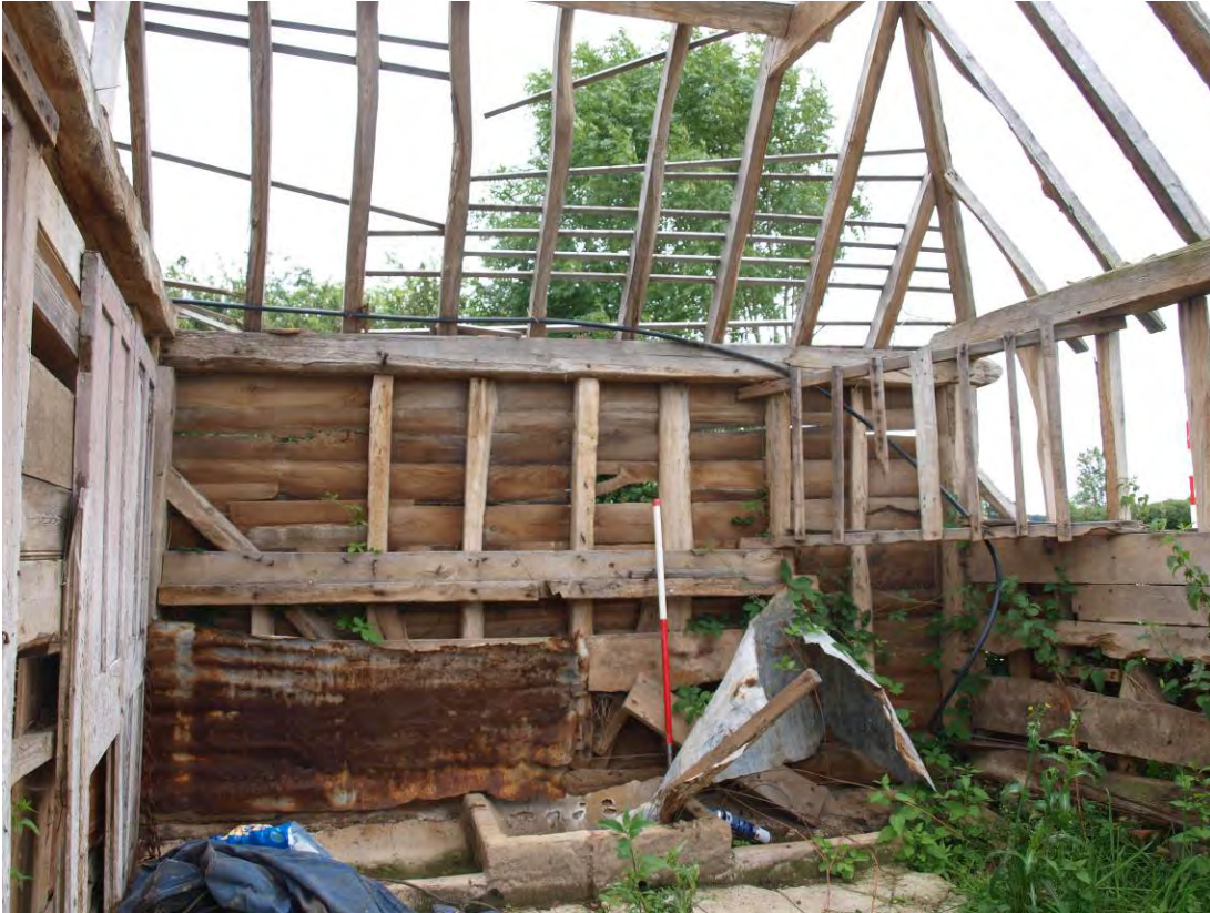
Plate 7: East wall of Bay 1 (Building 1), looking east
