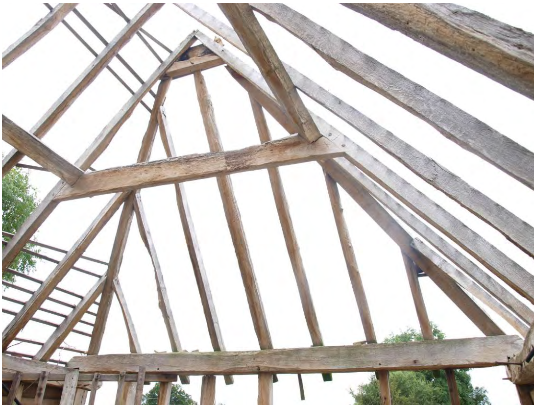
Plate 6: Hipped roof terminal to Building 1, looking south
