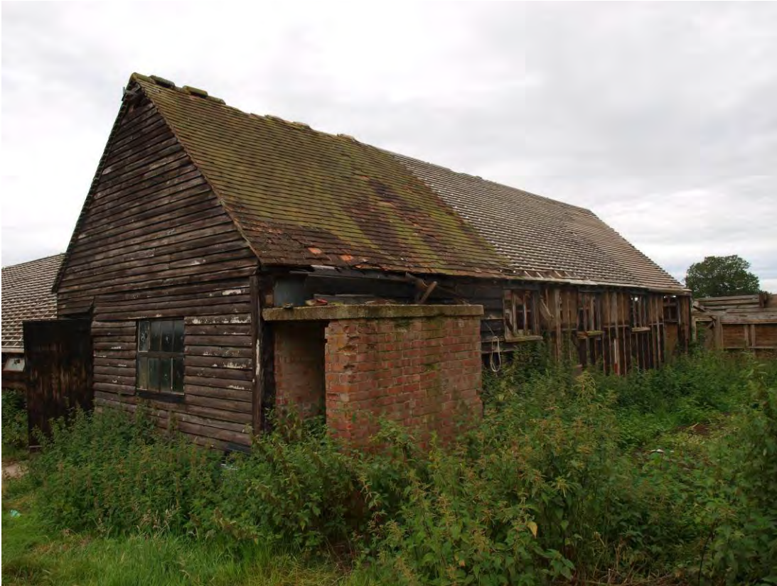
Plate 9: North and east elevations of Building 2, looking south-west
