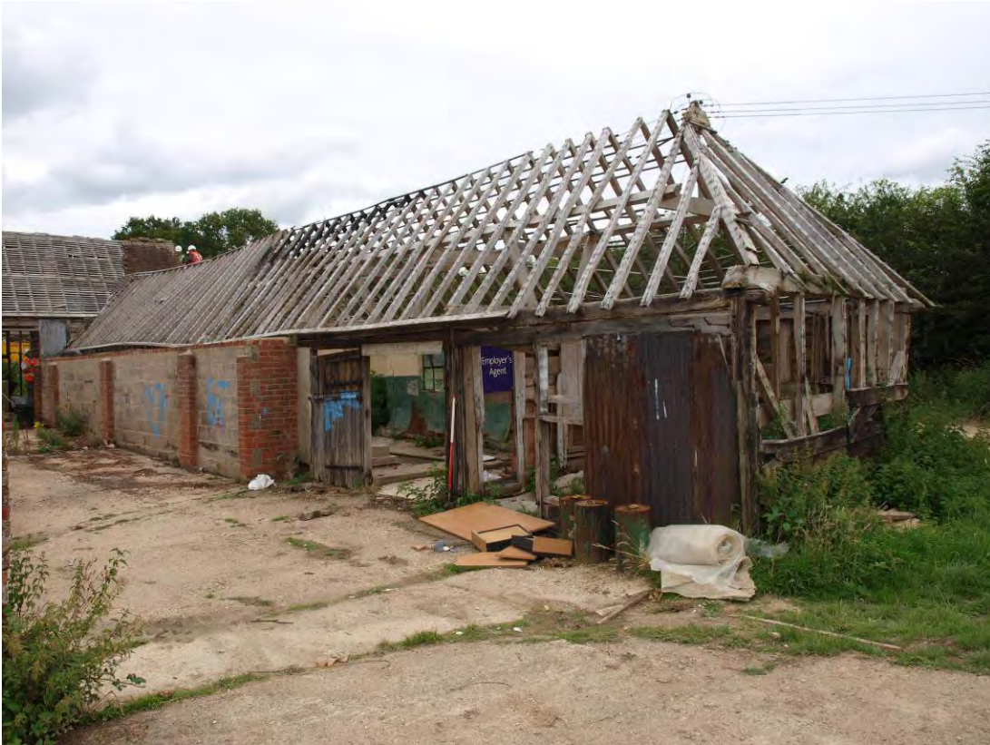
Plate 1: West elevation of Building 1, looking north-east
